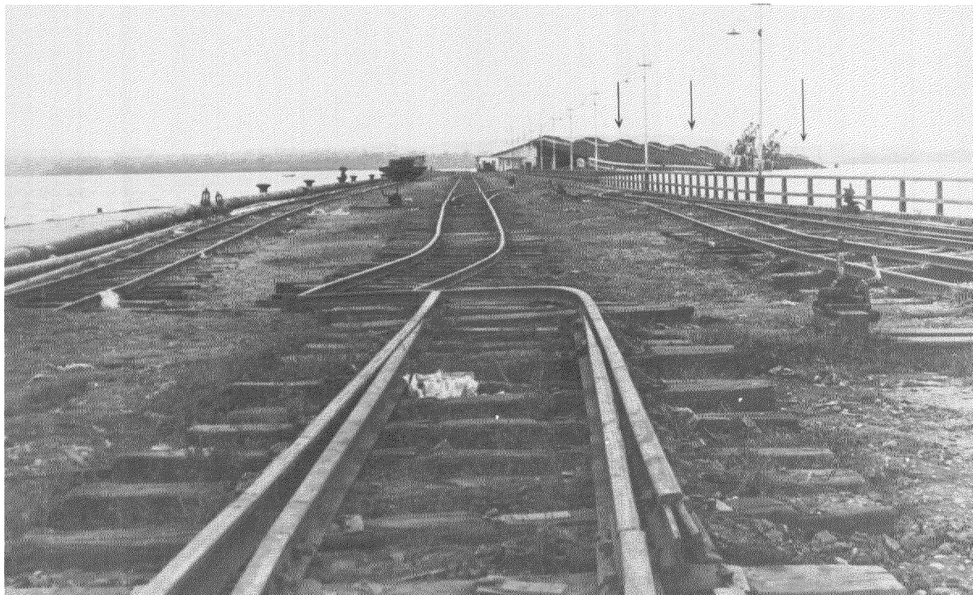
FIGURE 47.—Puerto Barrios wharf, Department of Izabal, destroyed by February 4 earthquake. Arrows show large warehouse partially submerged. See figure 40 for location of town.
