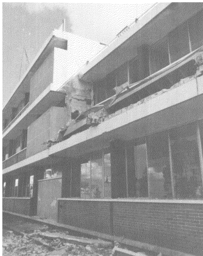
FIGURE 52.—Collapse of the second story of a building at the Colegio San Javier (Zone 12), Guatemala City.
