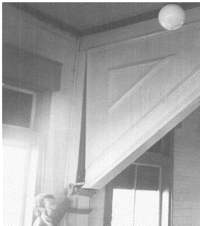
FIGURE 51.—Damage to a wooden structure in Puerto Barrios, caused in part by ground compaction. Note the large offset of 11 cm shown in the photograph.
