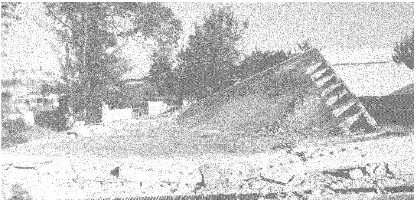
FIGURE 68.—Collapse of one-story reinforced-concrete framed structure in the Licorera Mixco, Mixco.
