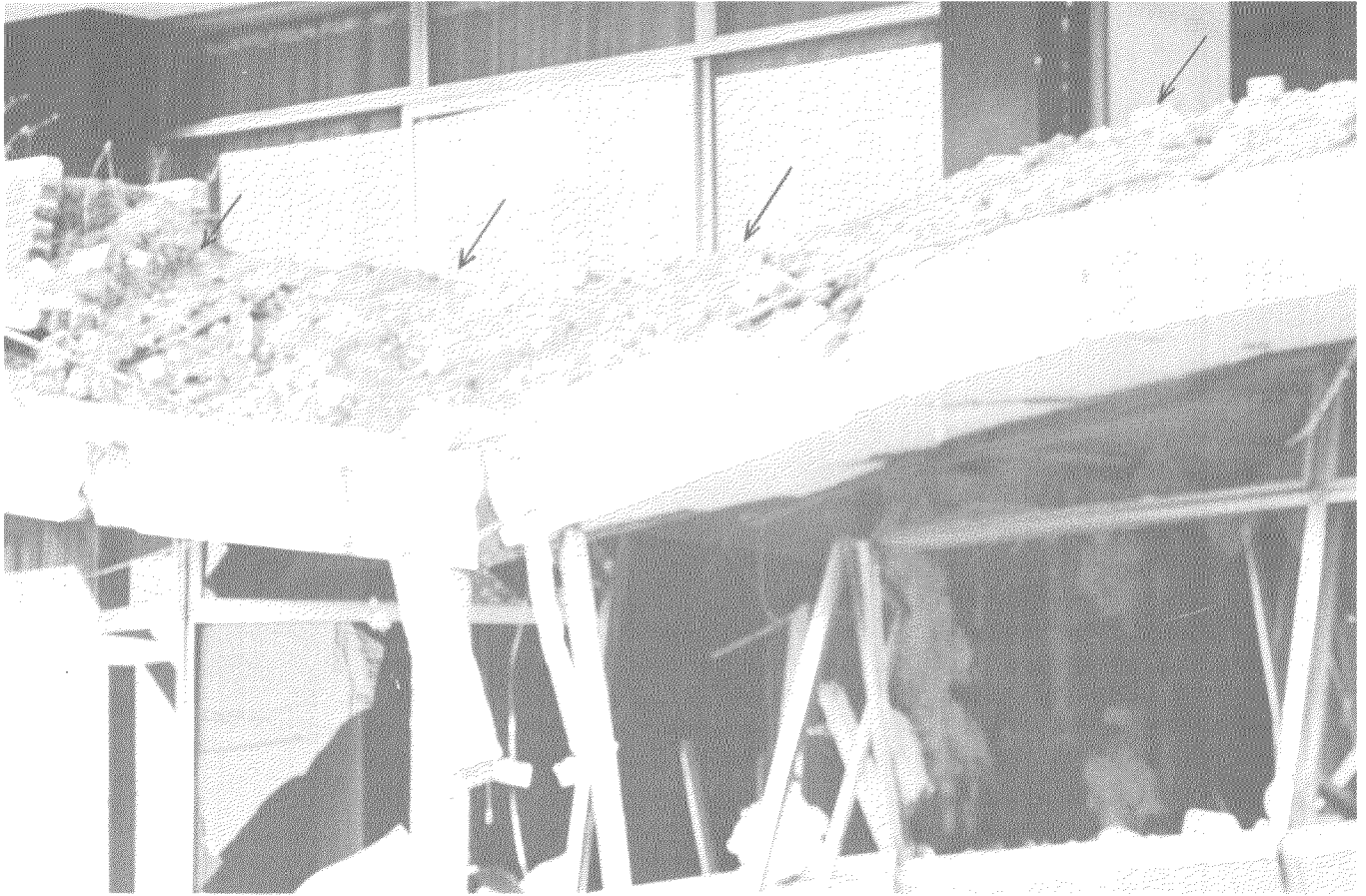
FIGURE 67.—Partial collapse of protruding first-story structure of the Cruz Azul 11-story reinforced-concrete building caused by falling (shown by arrows) of masonry walls from the two topmost stories, in Guatemala City (Zone 1).
