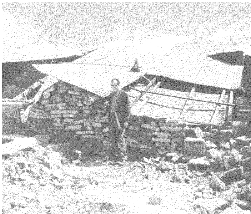
FIGURE 69.— A , Massive destruction of some adobe houses in Antigua, Guatemala, near the center of town. B , Large-scale destruction of adobe houses in Guatemala City, Calle 2 and Avenida 9A (Zone 2). C , Collapse of adobe houses in Guatemala City, Calle 22A and 34 Avenida (Zone 5). D , Collapse of adobe houses in Guatemala City, Calle 22 and Avenida 32 (Zone 5).
