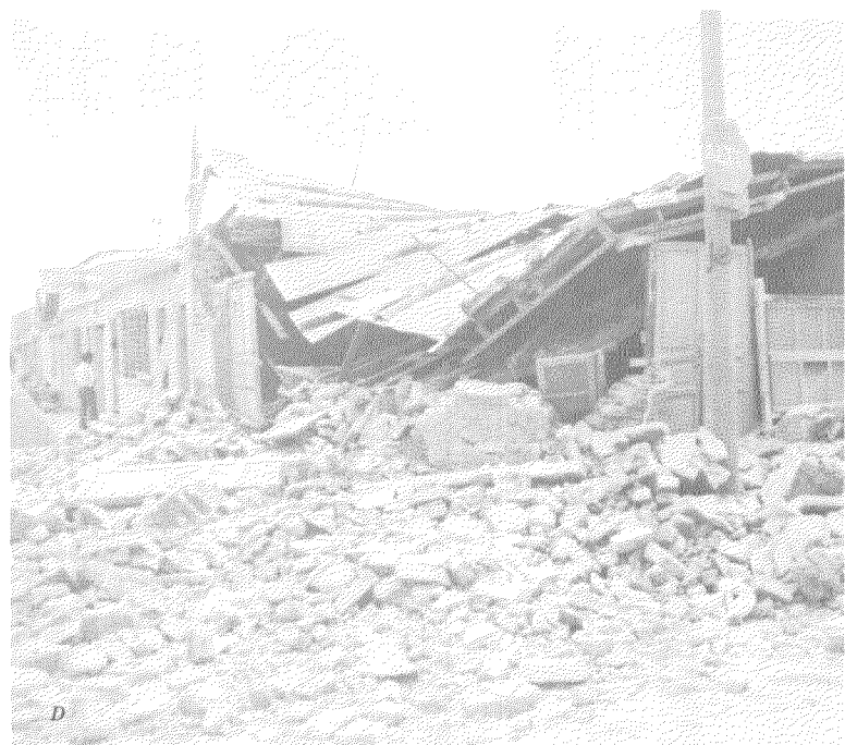
FIGURE 69.— A , Massive destruction of some adobe houses in Antigua, Guatemala, near the center of town. B , Large-scale destruction of adobe houses in Guatemala City, Calle 2 and Avenida 9A (Zone 2). C , Collapse of adobe houses in Guatemala City, Calle 22A and 34 Avenida (Zone 5). D , Collapse of adobe houses in Guatemala City, Calle 22 and Avenida 32 (Zone 5).
