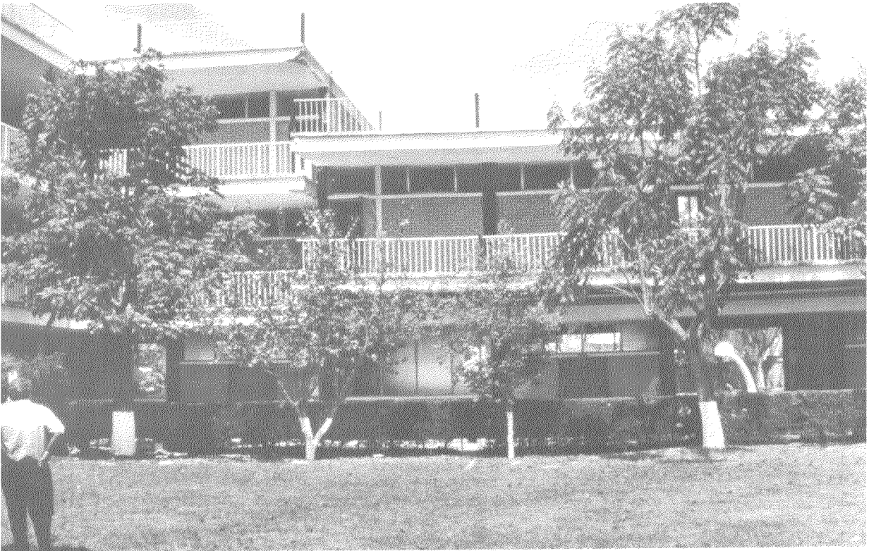
FIGURE 75.—Collapsed second story in one unit of the Catholic Boys School in Guatemala City. Roofs were originally at the same level.
