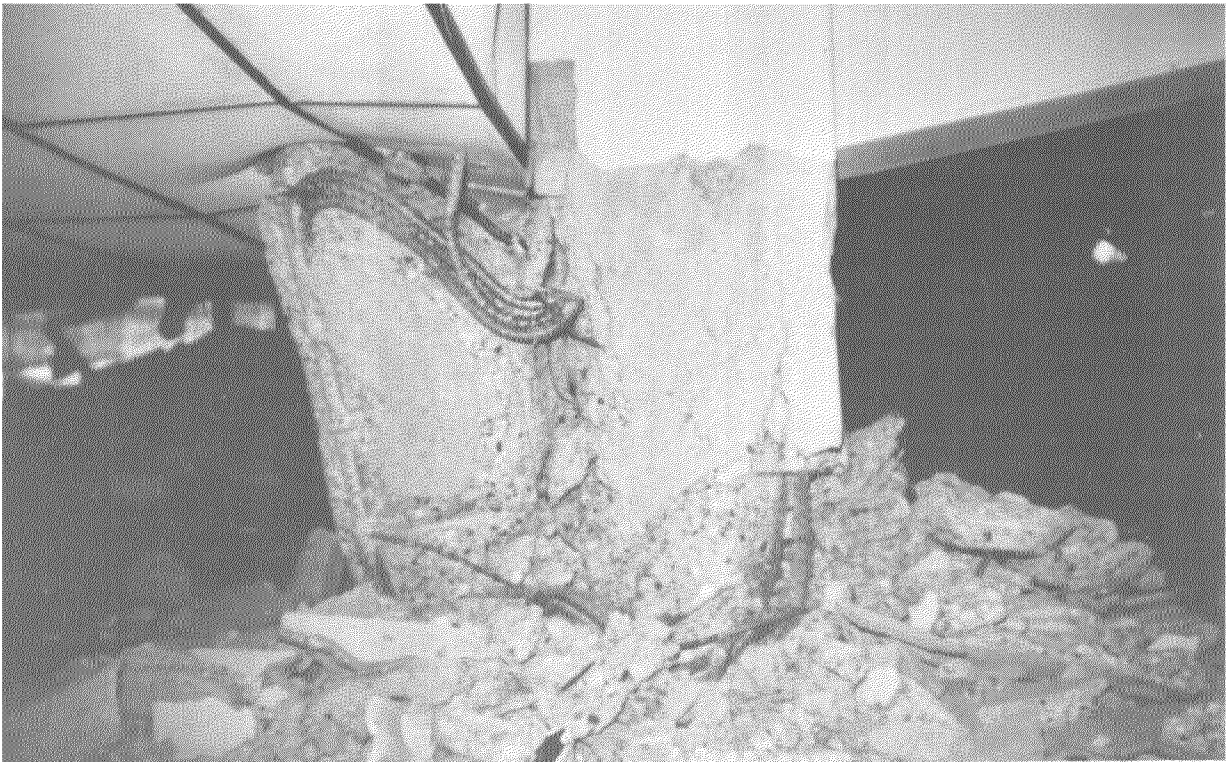
FIGURE 74.—Typical collapsed column in Hotel Terminal
