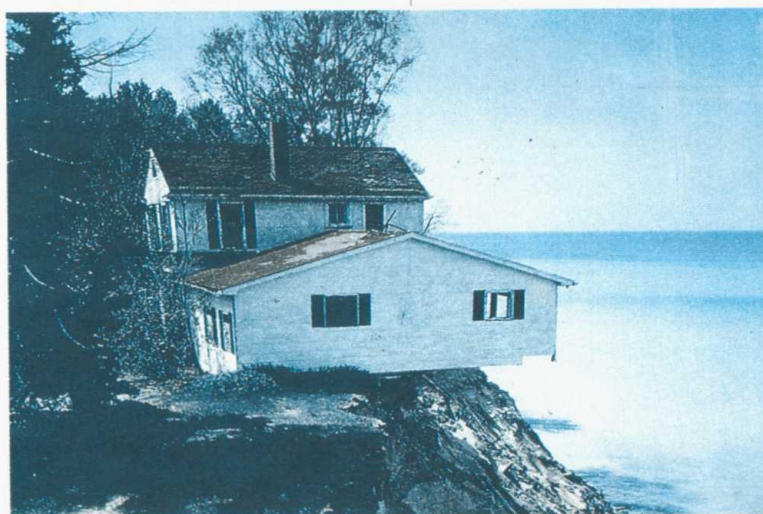
Landslide induced by coastal erosion. Courtesy: Australian IDNDR Co-ordination Committee.
