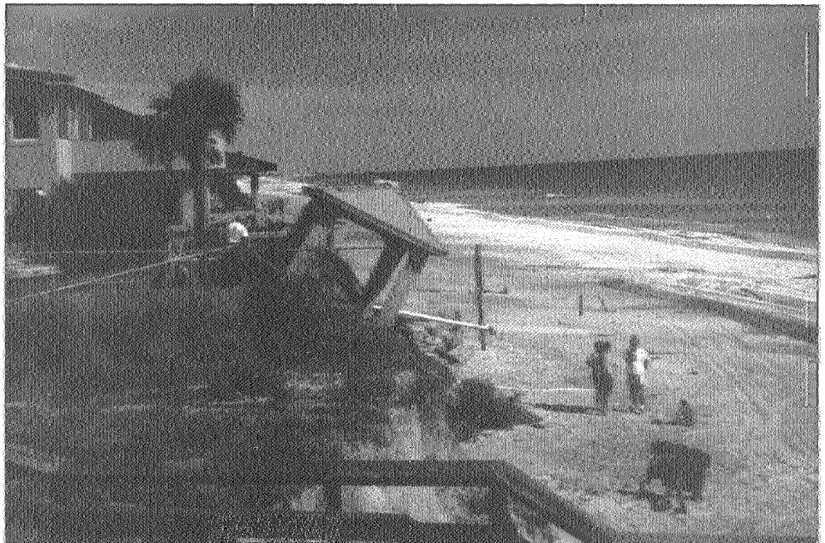
Figure 2-4 Erosion such as this took place along the gulf coast, causing structures to be undermined and resulting in damage.
