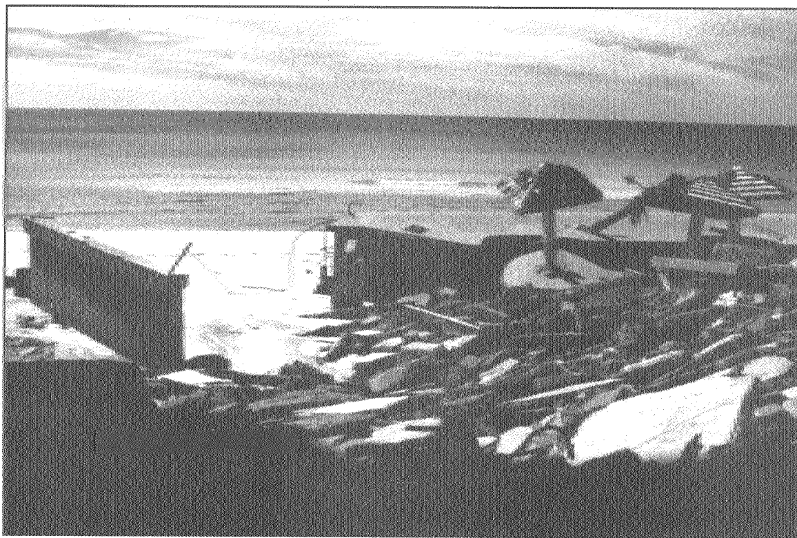
Figure 2-5 Debris, consisting of broken concrete and wood framing systems, generated by surge action
