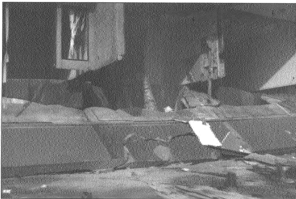
Figure 2-6 Undermining of concrete decks and floor slabs caused the failure of many unreinforced concrete structures.
