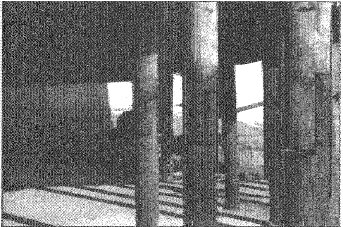
Figure 2-8 These piles were not long enough and were spliced to add depth. The splicing was exposed by storm-induced erosion.
