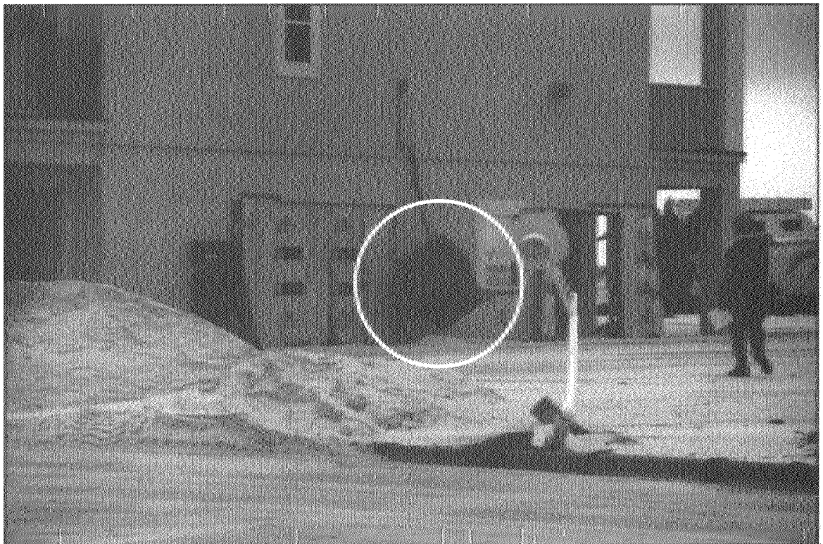
Figure 2-14 These breakaway panels functioned as designed. Note the loss of the air conditioning unit platform.
