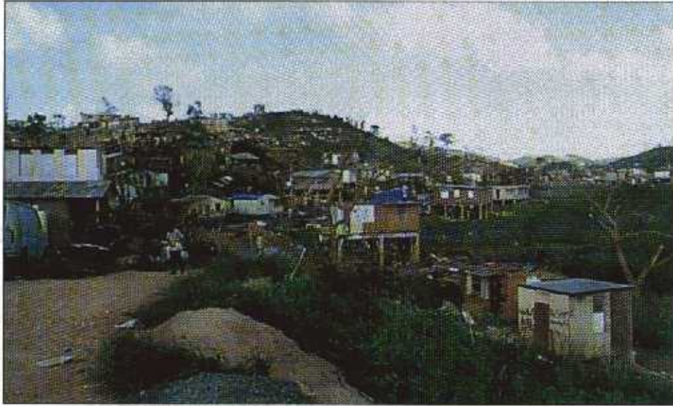
FIGURE 3-1 The abrupt change in topography in this community outside Loiza caused a speedup in the wind that flows over and around the buildings located on the hill beyond. The wind load provisions of Planning Regulation 7 did not account for wind speedup caused by abrupt changes in topography, and therefore underestimated wind loads on buildings situated on hills, mountains, or escarpments.
