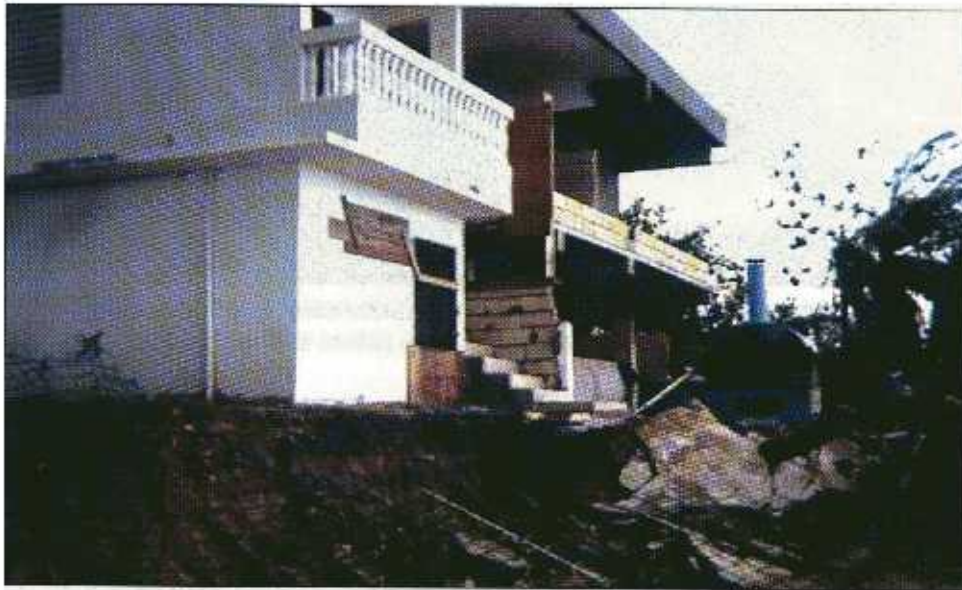
FIGURE 3-9 Structure along the coast damaged by storm surge and wave action.
