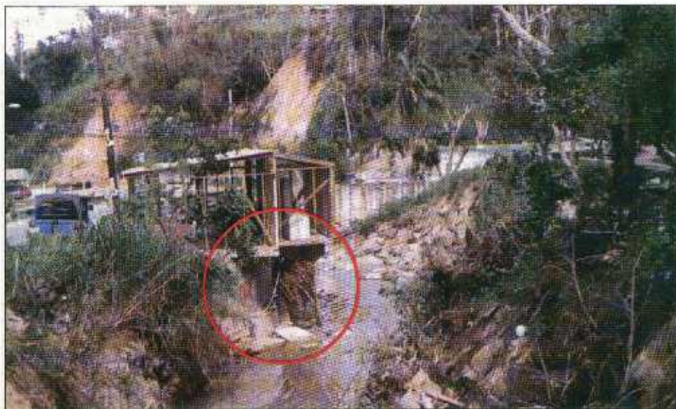
FIGURE 3-8 Typical construction adjacent to and over the river. Note the debris trapped under the concrete foundation and between the framing.
