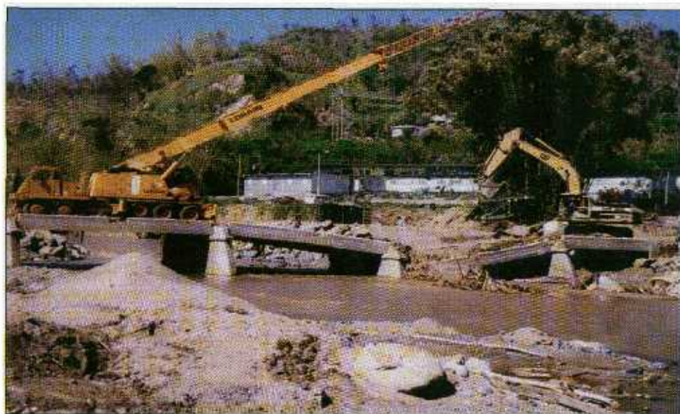
FIGURE 3-12 This bridge outside Adjuntas collapsed due to insufficient design to resist the effects of floodwaters.
