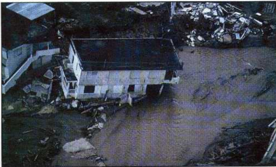
FIGURE 3-6 Floodwaters eroded soil and undermined the foundation system of this building.
