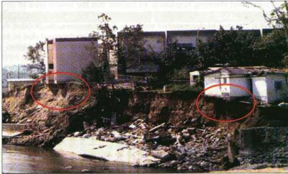
FIGURE 3-7 Riverbank erosion resulted in the undermining of the building foundations of a school (pink building) and house (white building) in Jayuya.
