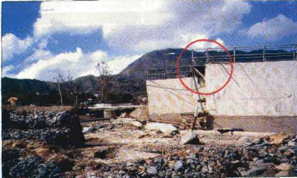
FIGURE 3-13 Severely damaged water treatment facility located in the floodplain in Jayuya; floodwaters overtopped the concrete wall.
