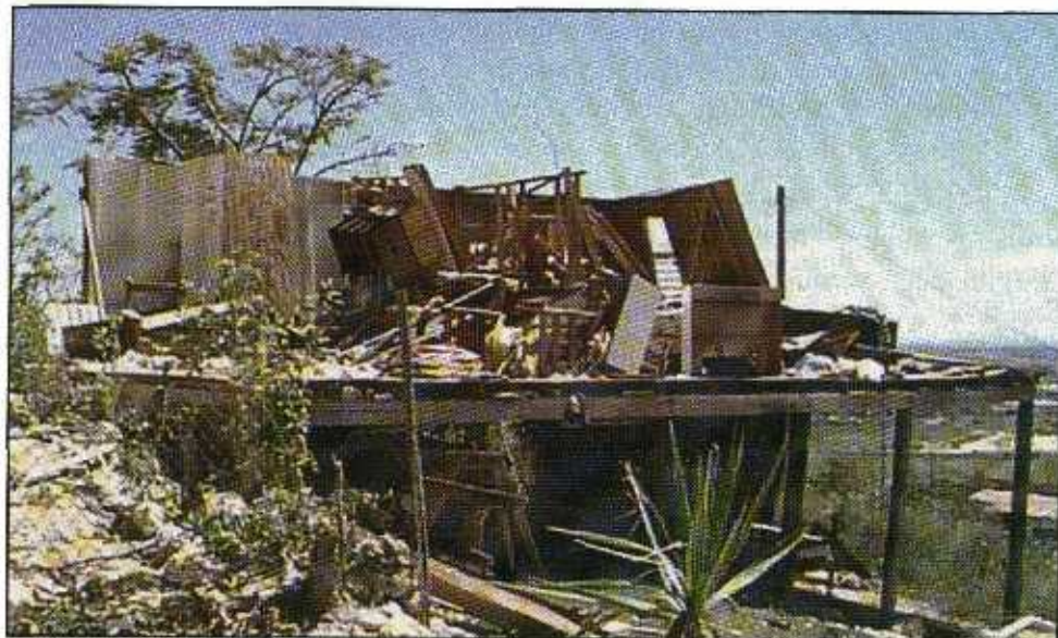
FIGURE 3-23 A residential wood structure located on the hilltops west of Ponce destroyed by wind. The roof system has been removed and the wall system partially collapsed.
