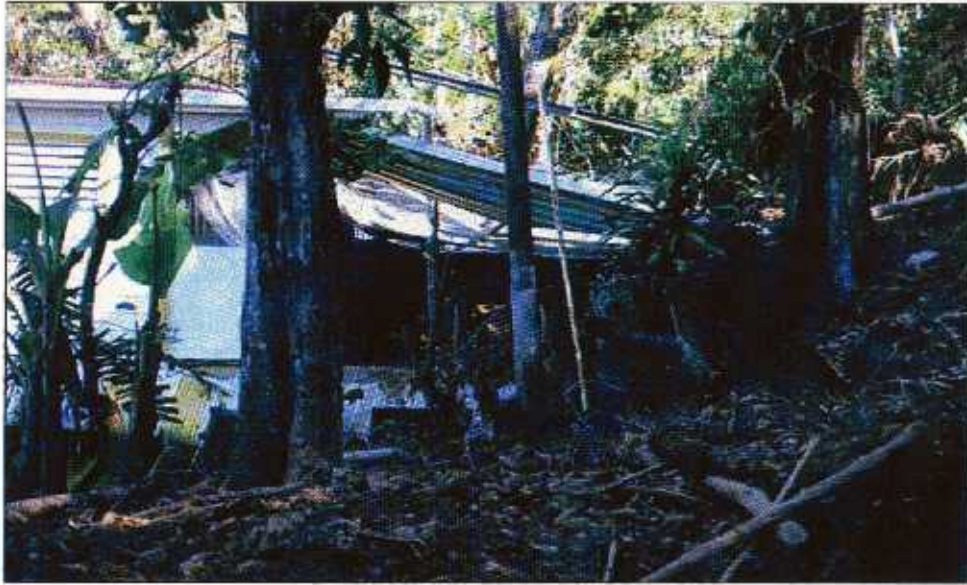
FIGURE 3-15 A landslide inundated this house with up to 5 feet of soil.
