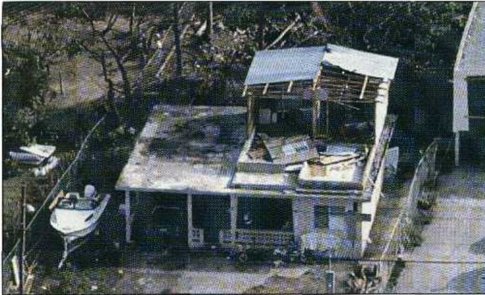
FIGURE 3-21 A combination residential concrete/masonry structure with an elevated second-floor concrete slab and a wood-framed upper level. Note the lack of damage to the concrete/masonry section of the house and the damage to the wood-frame portion.
