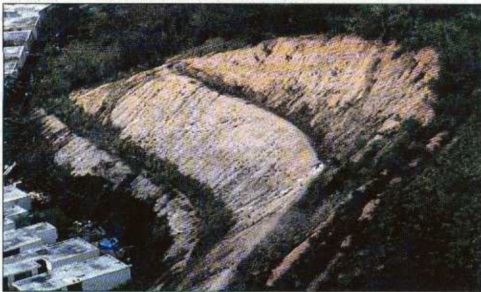
FIGURE 3-16 Development adjacent to a representative unprotected cut; the potential for future landslide activity exists.
