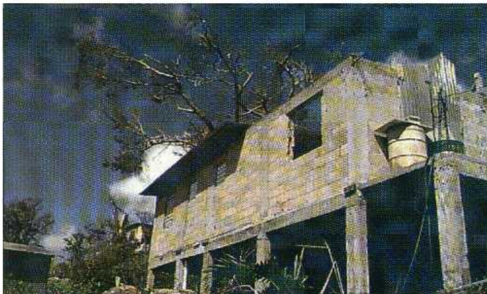
FIGURE 3-22 A residential concrete/masonry structure that is under construction. The photograph illustrates this common building practice: concrete columns with unreinforced masonry block infill walls. This is not seismic resistant construction.
