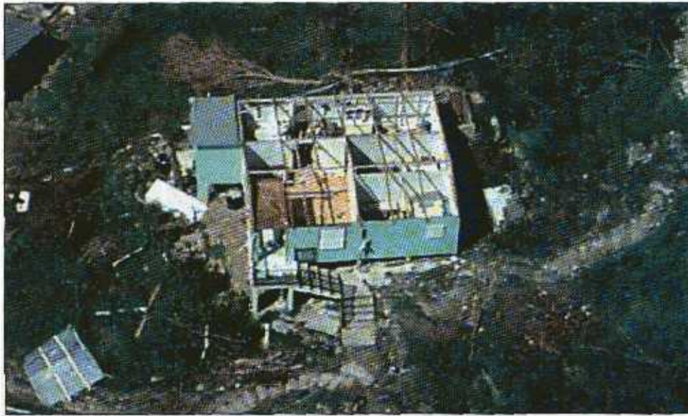
FIGURE 3-20 Aerial view of a residential concrete/masonry structure with a wood-frame roof structure; only the roof rafters remain. The wood nailers and metal panels were blown off.
