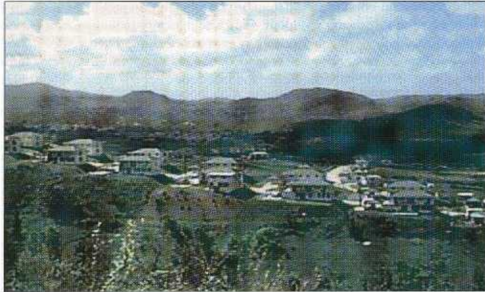
FIGURE 4-2 A residential community constructed of concrete and masonry buildings with concrete roof structures. This community, located to the west of Luquillo experienced no complete building failures. The eye of the hurricane passed to the south of this community, placing it in the strongest wind quadrant of the hurricane.
