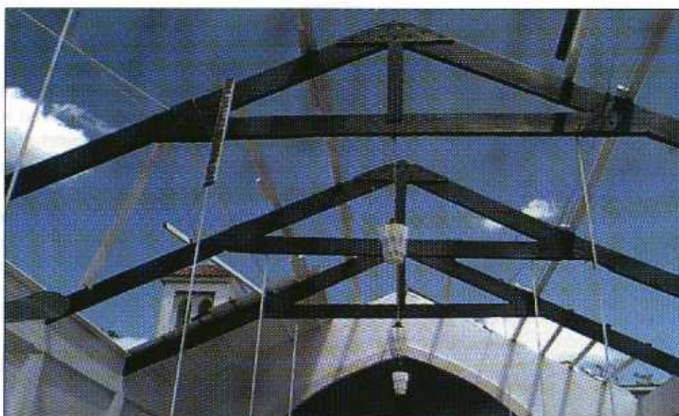
FIGURE 4-9 Masonry wall church that lost roof purlins and its corrugated metal roof. Nails were the only connections used to resist wind loads. The gable ends of this church were unsupported except for purlins resting in the masonry.
