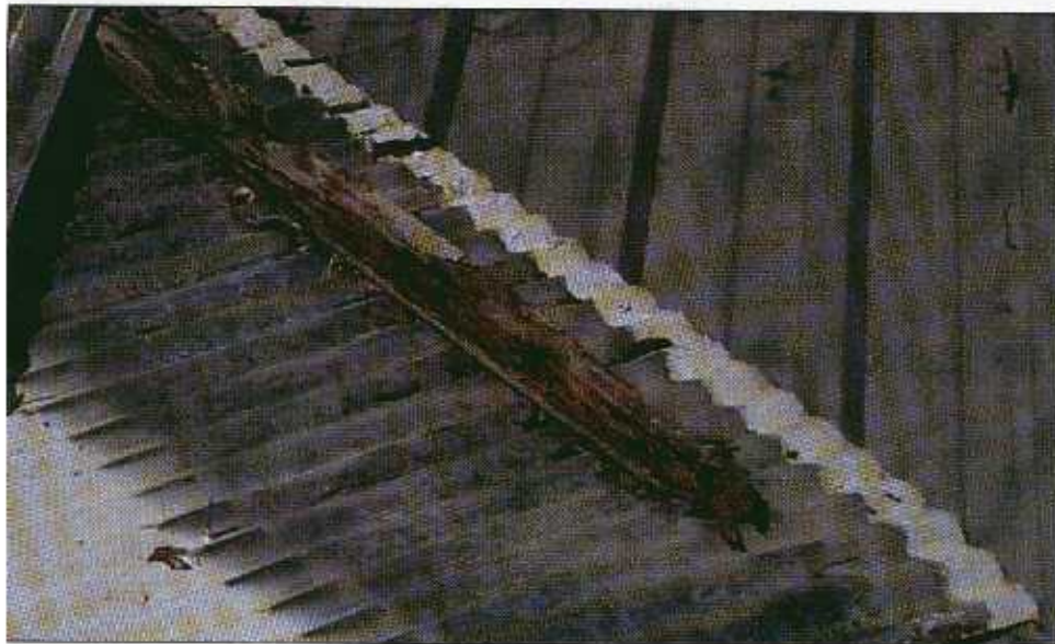
FIGURE 4-8 Termite-damaged wood purlin attached to metal roof panel. The entire roof system of this building failed and is shown in Figure 4-9.
