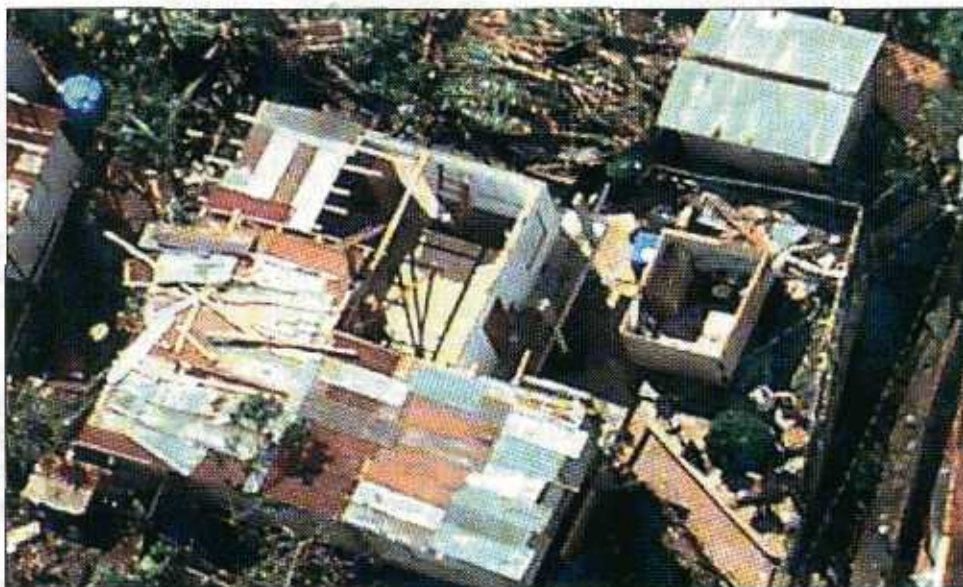
FIGURE 4-7 Typical roof system failure between wooden roof system and concrete or masonry wall system.
