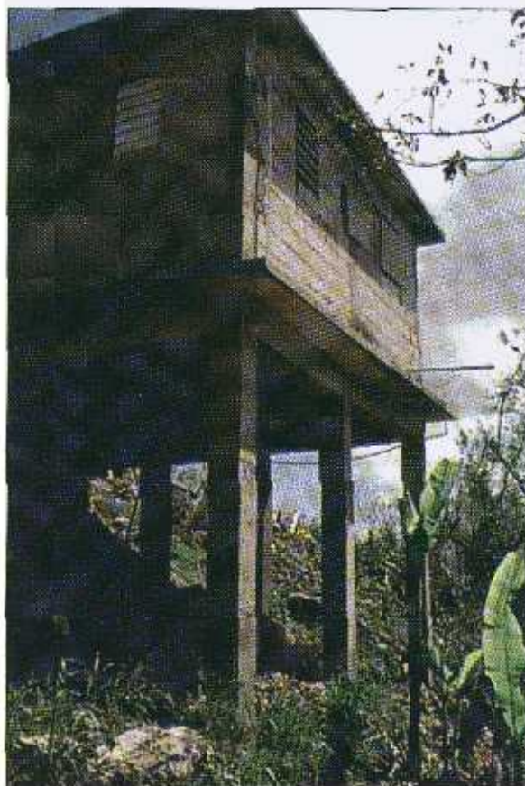
FIGURE 4-22 Residential building supported atop tall, unbraced concrete columns. This type of unbraced support column was common in many areas.
