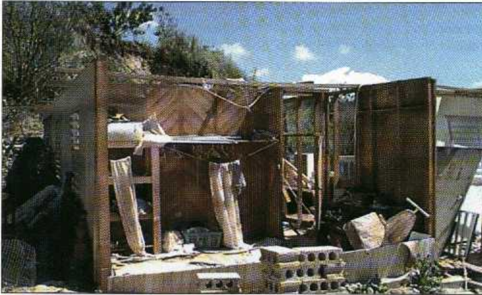
FIGURE 4-14 Example of wood-frame wall construction that failed during Hurricane Georges. This building was not constructed with any hurricane clips or straps.
