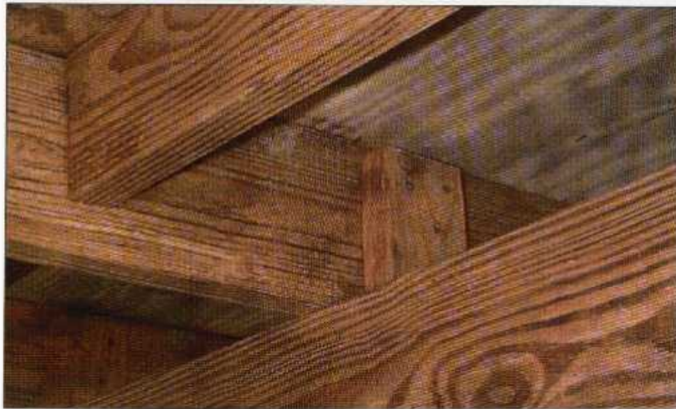
FIGURE 4-20 Example of a successful wood connection between support beam and floor joists. This is the same house shown above in Figure 4-19.
