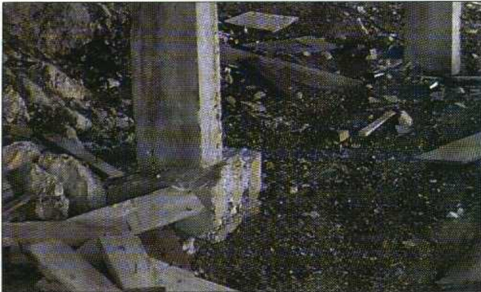
FIGURE 4-23 Footing for tall columns in Figure 4-22. This footing is not adequately anchored to the supporting rock to resist lateral forces that may be induced during a design seismic event.
