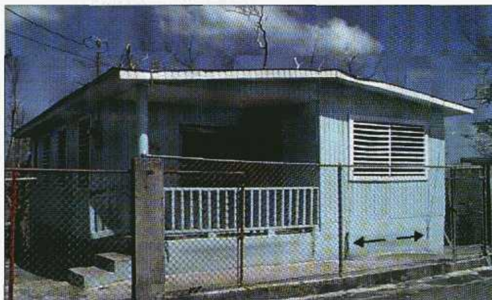
FIGURE 4-21 Wood-frame house with metal roof covering with hold-down cables that run parallel (see arrows) and perpendicular to the roof ridge line. This house was set atop a ridge that experienced significant winds. The lack of damage can be attributed to the extra care taken in fastening down the corrugated metal roofing. The strapping would not have prevented buckling of the roofing or uplift at the eave.
