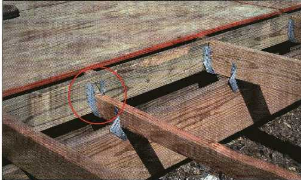
FIGURE 4-13 Example of the failure of wood member in the floor joist hanger due to the use of improper nails. The hurricane clip was used to secure the floor joist to the support beam. This house was located on the island of Culebra.
