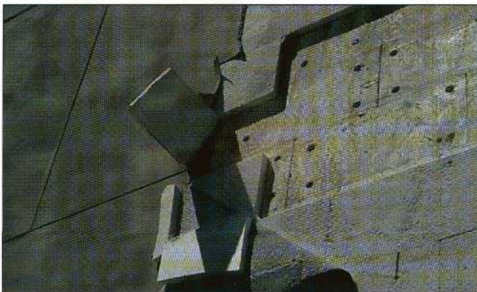
FIGURE 5-11 At this EIFS covering, the synthetic stucco appeared to be well-adhered to the outer EPS layer, but there appeared to be minimal bonding between the two EPS layers. In at least the lower portion of the wall, the first layer was attached with mechanical fasteners deeply recessed into the foam. The delamination occurred near the corner of the building, where the suction pressures were high.
