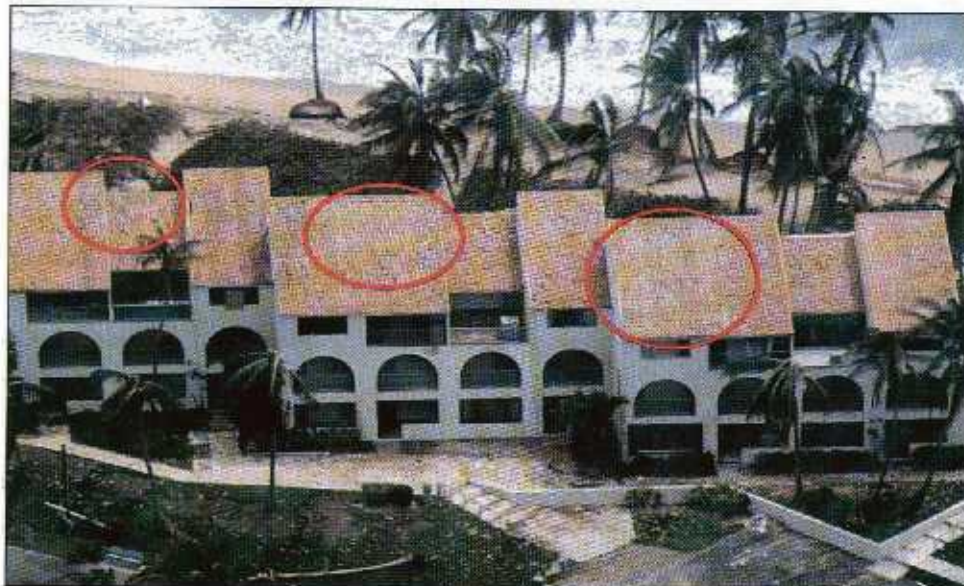
FIGURE 5-20 These tiles were heavily damaged, although the wind speed at this location was not very high. As can be seen in the foreground, the roof covering generated a substantial number of missiles. Because of the relatively low wind speed, the tile debris did not travel very far.
