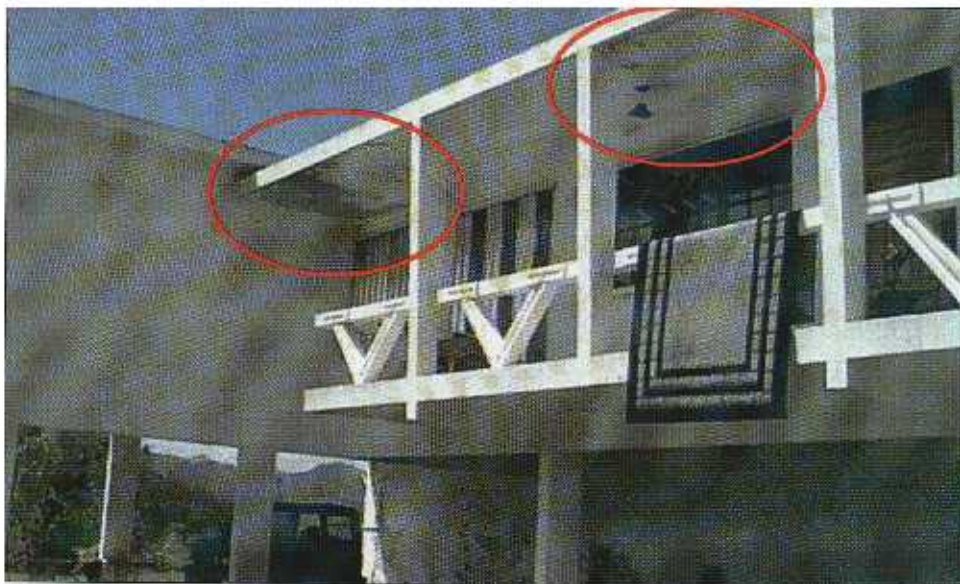
FIGURE 5-13 This house was located on a mountain top that experienced very high wind conditions. The paint scoured off at some of the soffit areas and along the recessed wall.
