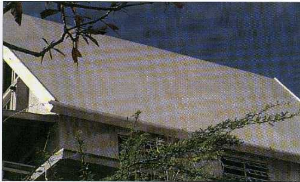
FIGURE 5-21 This house had a liquid-applied membrane over plywood roof sheathing. This type of roof system typically offered excellent wind performance provided the plywood does not lift. This house was located on the island of Culebra.
