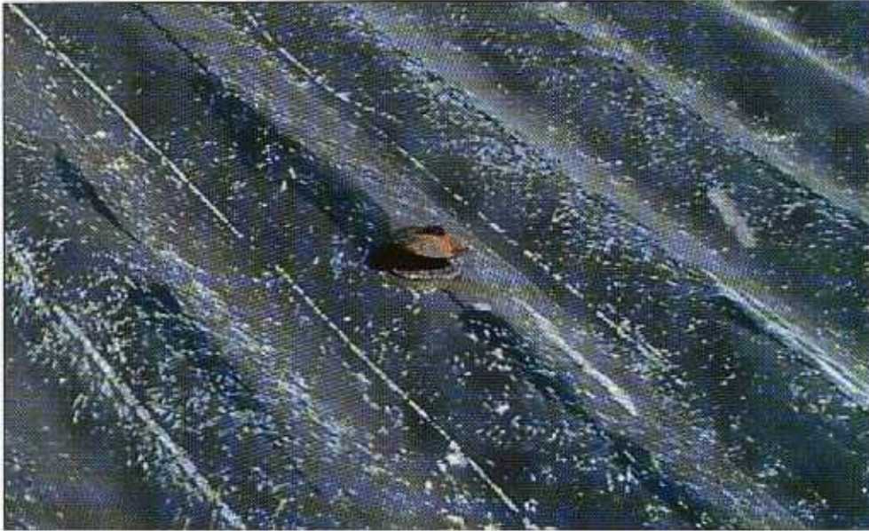
FIGURE 5-14 The nail attaching this corrugated metal panel partially backed-out. Screws are much more resistant to back-out. Nail back-out is a problem with metal panel systems because of the large number of load cycles and large amount of deformation the panels can experience during a hurricane. Elsewhere on this roof, some of the panels were blown off.
