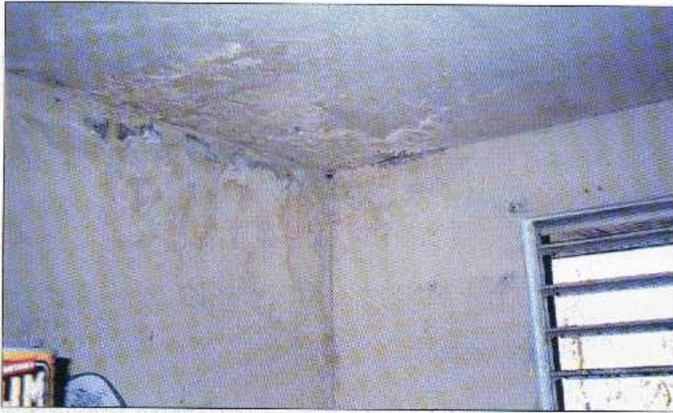
FIGURE 5-19 This concrete roof deck did not have a roof covering. During the hurricane, water entered the house through the deck. The concrete deck and CMU walls were skimmed with a skim coat of plaster. This house has Miami windows.
