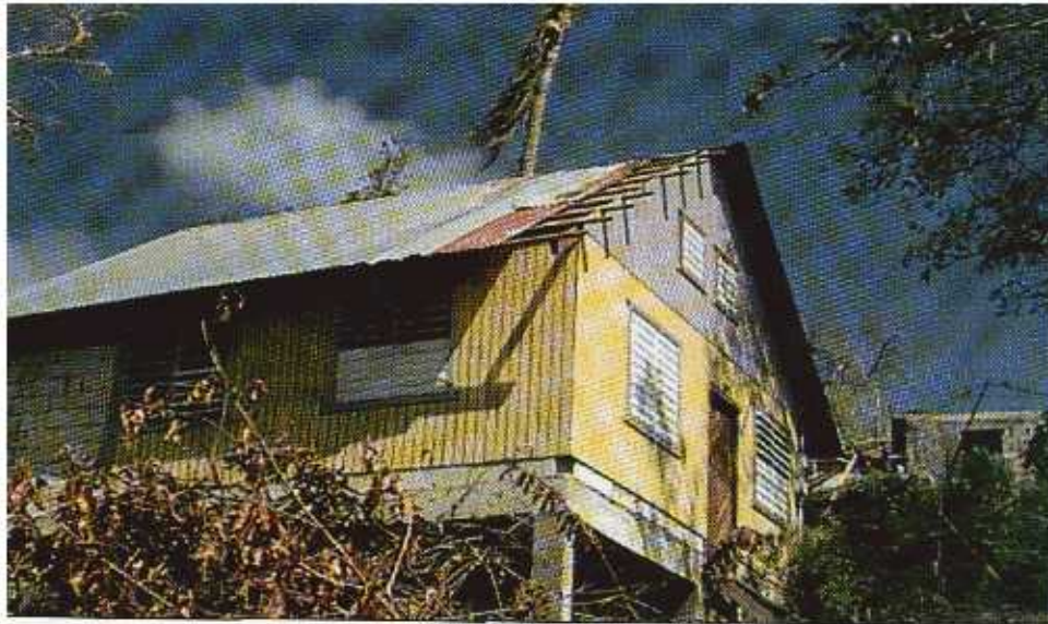
FIGURE 5-16 The metal panels along this rake were insufficiently fastened. A framing member was not run up the rake.
