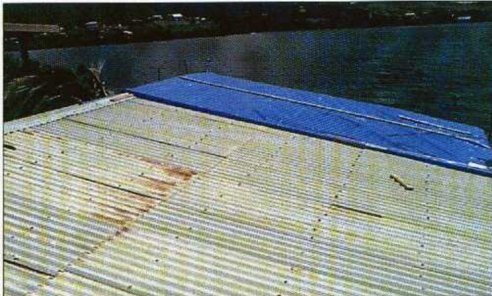
FIGURE 5-15 Only a single row of fasteners were installed along the eave and along each side of the ridge. The side laps are insufficiently attached and are lifting in a few areas. The end lap is too far away from the first row of fasteners—another nailer should have been installed. Clips between the joists and wall were retrofitted prior to the hurricane; however, enhanced attachment of the metal roofing was not performed as part of that work. As a result, several of the metal panels were blown off.
