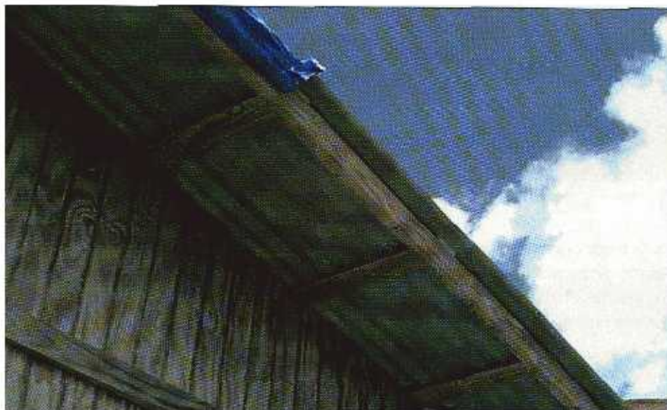
FIGURE 5-17 At this house, a framing member was run up the rake, which allowed the metal panels to be fastened between the nailers (purlins). However, the rake member must have sufficient strength to resist design uplift loads, which does not appear to be the case with this member. Rather than installing a metal edge flashing, these metal panels simply were cantilevered beyond the rake framing, providing a loose edge that is susceptible to lifting and peeling during high winds. Other deficiencies that are noted in this photograph include incorrect nailing of roof material to rake member and inadequately sized and spaced nailers.
