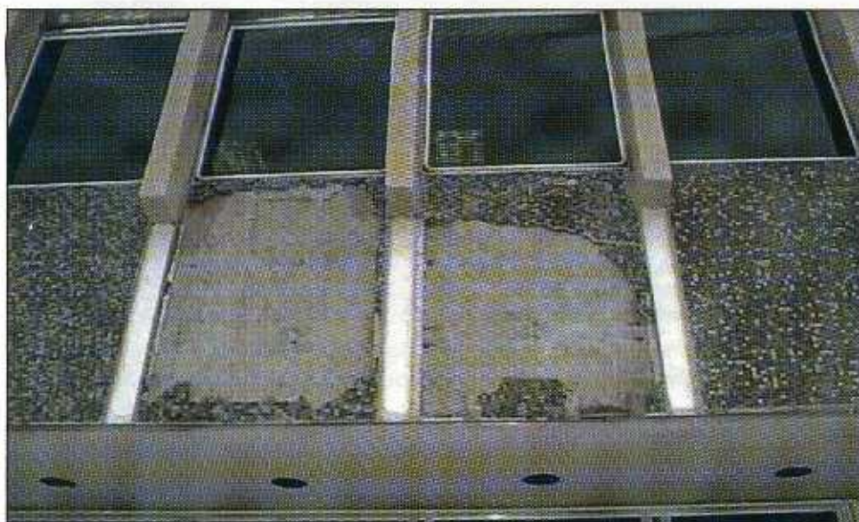
FIGURE 5-12 A mortar skim coat was applied over the concrete, and the ceramic tiles were set in to the mortar. The primary failure plane was between the mortar and concrete.
