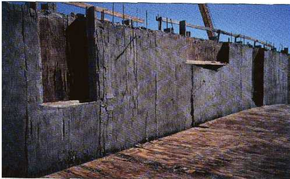
FIGURE 5-10 This house is under construction. The surface of the concrete is very rough because the plywood form (which is lying down on the ground) was used repeatedly. The rough texture will be compensated for with a stucco surfacing.
