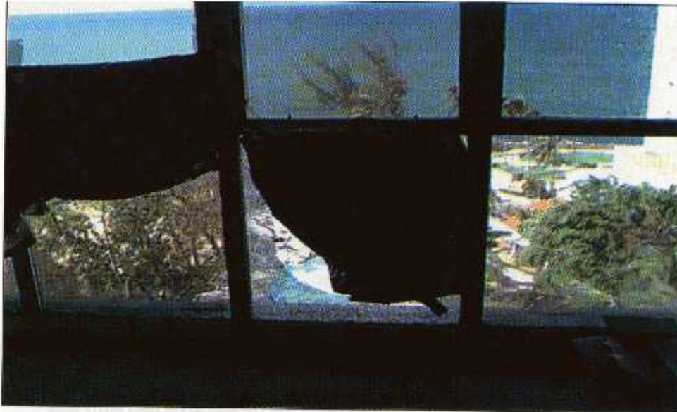
FIGURE 5-24 When these tempered panes broke, they did not produce shards of glass, as did the annealed panes.
