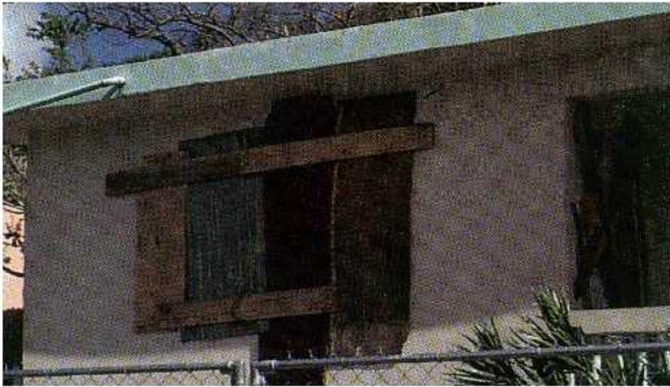
FIGURE 5-33 A combination of boards and metal panel was used to construct this shutter. Unless shutters are well attached, they can blow off during high winds and become missiles themselves.
