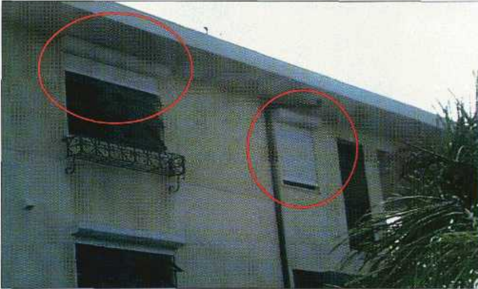
FIGURE 5-37 These windows were equipped with roll-up shutters.
