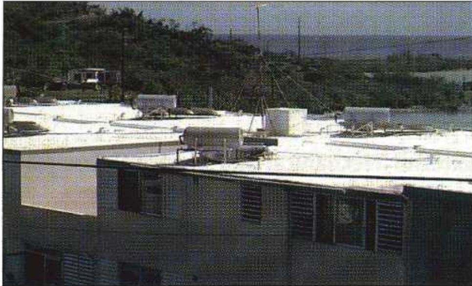
FIGURE 6-2 This roof had several solar hot water heaters that successfully weathered Hurricane Georges. However, the unit in the foreground was damaged.
