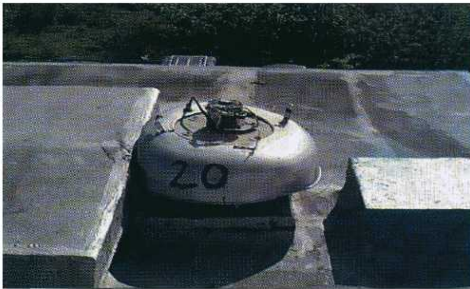
FIGURE 6-1 This exhaust fan lost its cowl.
