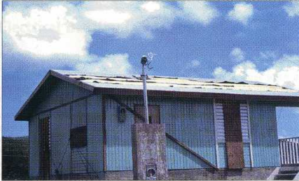
FIGURE 6-4 This service mast is mounted on a concrete pylon. This form of service connection was successful in eliminating roof damage when the overhead service blew down.
