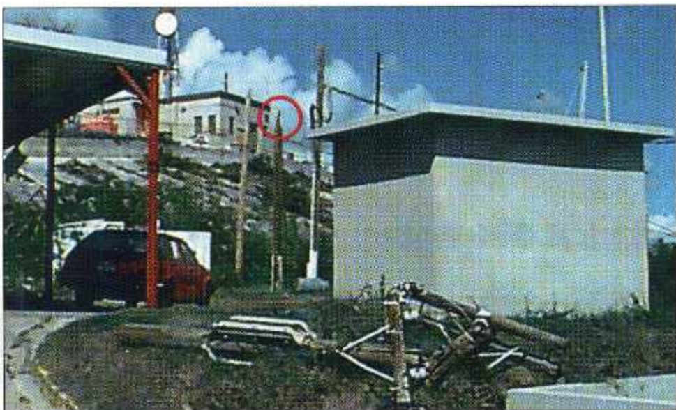
FIGURE 7-1 Damaged wood pole. The portion of the wood pole in the foreground broke from the pole (circled) in the back of the picture.
