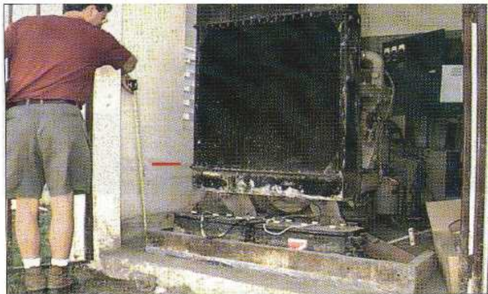
FIGURE 6-3 Flood water entered this generator room and reached a height of about 2 feet, as indicated by the red line. This facility is located in Jayuya.
