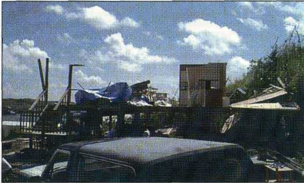
FIGURE 8-2 This wood-framed house was nearly totally destroyed. This is in remarkable contrast to the nearby building shown in Figure 8-3.
