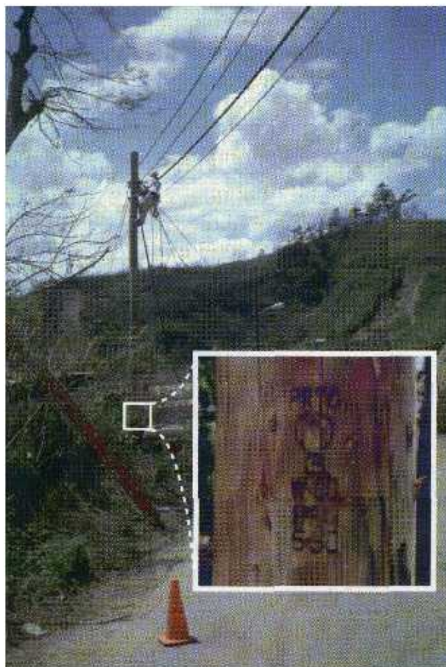
FIGURE 7-4 New wood pole replaced after the hurricane; utility lines are still being attached to the pole. Inset shows wood pole grade marking. This #3 pole was typical of those used throughout the island.
