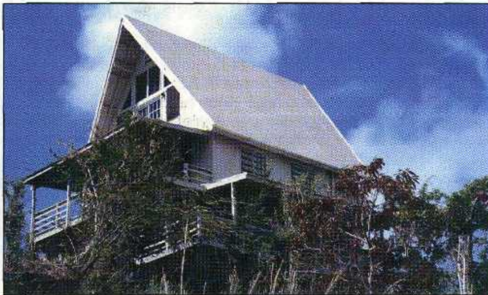
FIGURE 8-3 This wood-framed house is close to the house shown in Figure 8-2. The wind flow was essentially identical at these two sites, hence the successful performance of the one building is attributable to the attention given to design and construction. The value of mitigation is clearly illustrated in these two starkly different cases.
