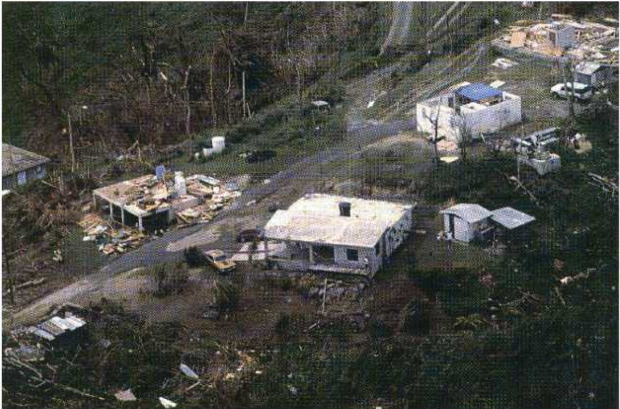
FIGURE 9-1 This photograph illustrates successes and failures in residential buildings observed after Hurricane Georges. A residential concrete building with no structural damage is seen in the center of the picture. At top right is a wood-frame building that is completely destroyed around a center room that was constructed of masonry. Other buildings in the photograph have damage that ranges from the total loss of the wood-frame building to the success of the concrete building.
