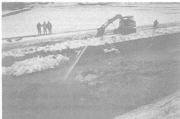
Photo.3 Cleaning operations using a high pressure pump (March 9)
