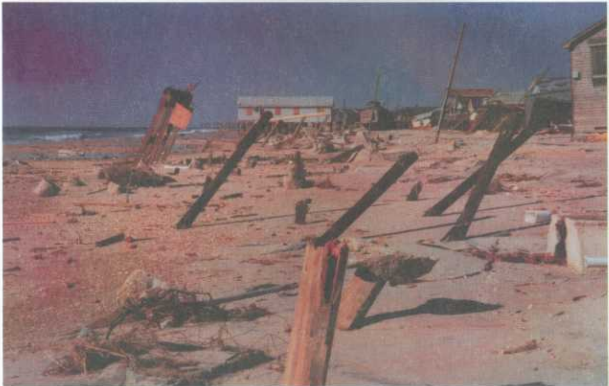
Figure 2-4 Loss of the frontal dune and the resulting erosion and scour left many coastal houses unable to resist wind and flood loads acting simultaneously.
