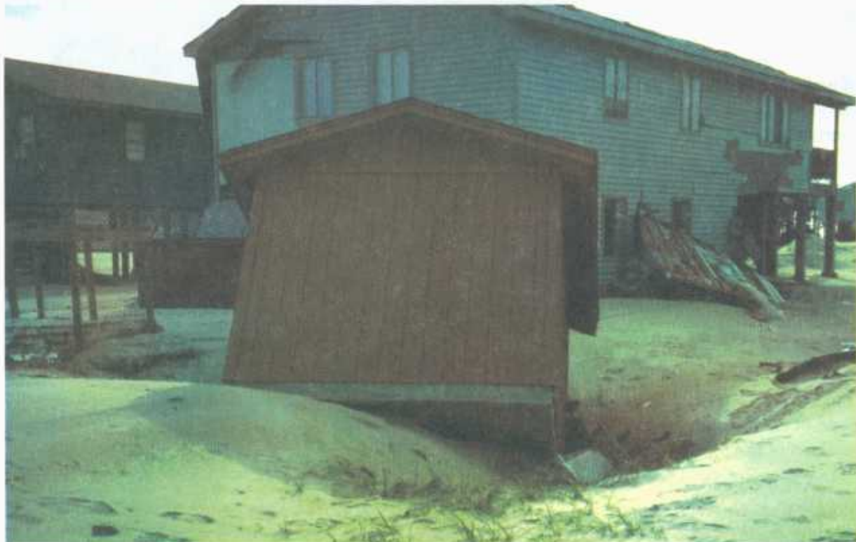
Figure 2-5 Overwash of barrier islands generated high-velocity flows that caused extensive scour adjacent to large objects.
