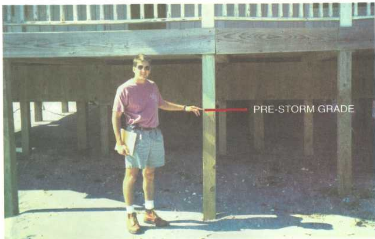
Figure 2-2 Erosion resulted in significant loss of supporting sand, averaging 4 to 6 feet, under oceanfront buildings.
