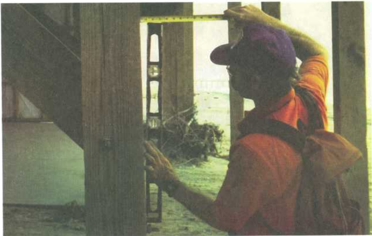
Figure 2-10 One of several buildings observed to be leaning landward that were suspected of having been constructed to current North Carolina State Building Code requirements.
