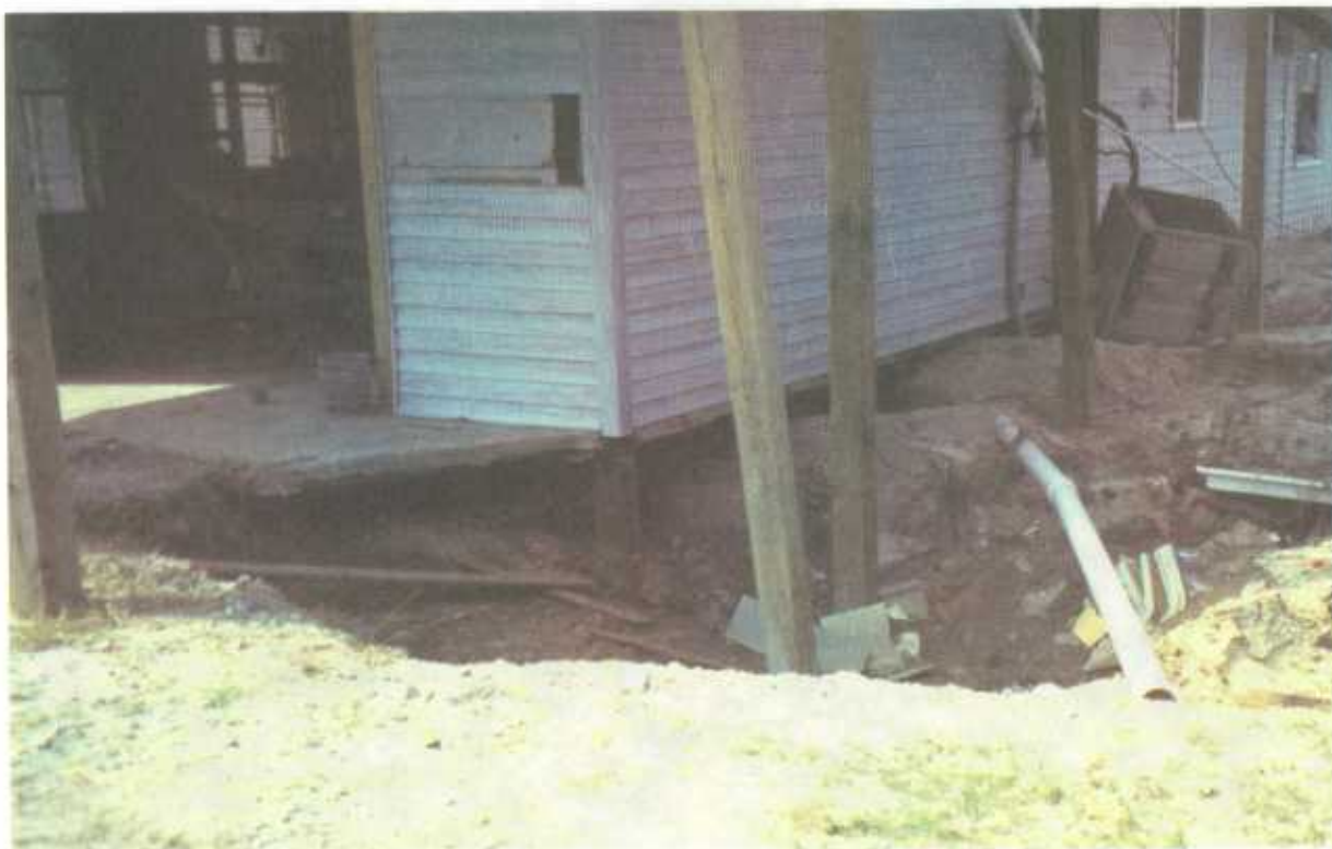
Figure 2-6. The disruption of velocity flows by large, non-breakaway objects generated extensive scour that undermined vertical foundation members and slabs-on-grade.
