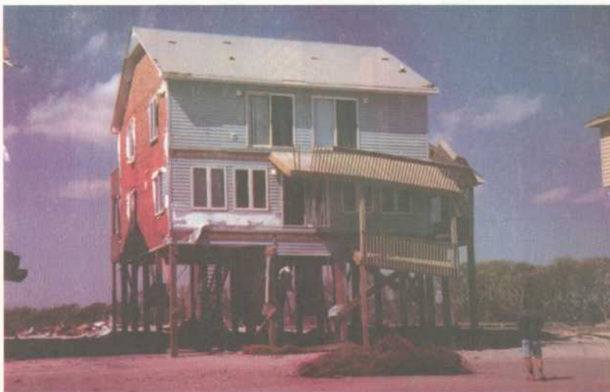
Figure 2-11 The BPAT observed several hundred decks and porches that collapsed as a result of insufficient foundation support.
