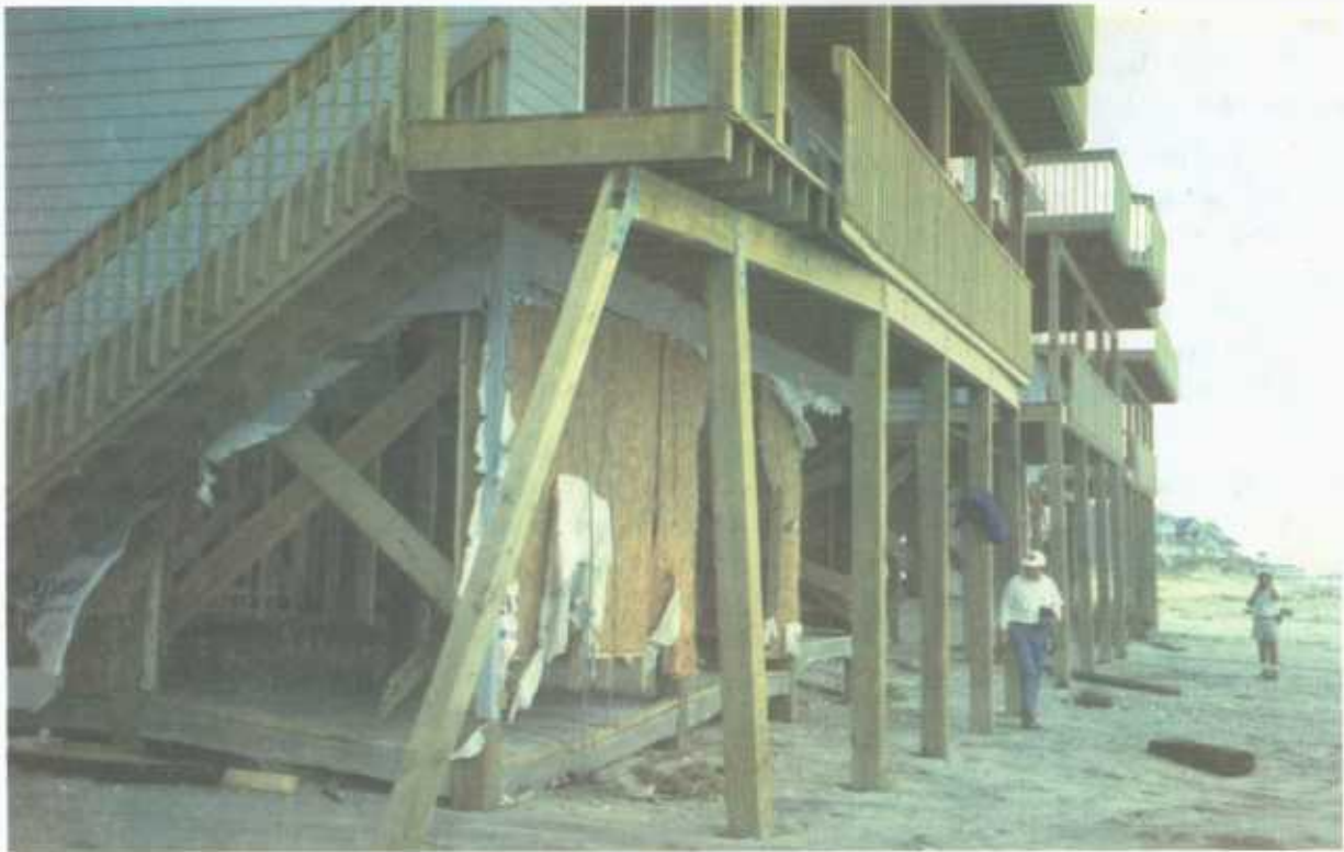
Figure 2-12 Example of building constructed to current North Carolina State Building Code requirements with insufficient embedment of piles/columns under two-story deck.
