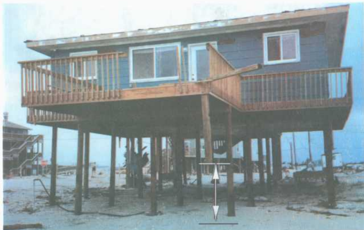
Figure 2-13 Embedment of deck supports into frontal dune was often shallow. After erosion of the dune, the bottom of the support for this deck was left several feet above grade.
