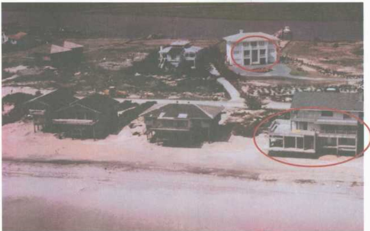
Figure 2-15 As shown by this post-Fran photograph taken at Figure Eight Island, North Carolina, a current architectural trend is the construction of multistory decks supporting roof overhangs.
