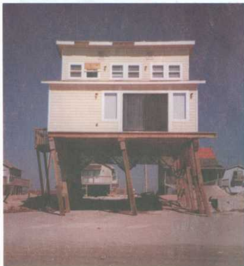
Figure 2-8 Many oceanfront houses built prior to current (1986) North Carolina State Building Code requirements were found to be leaning or destroyed.
