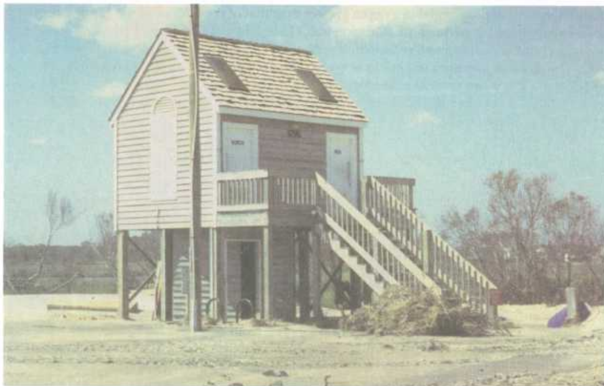
Figure 2-21 Survival of this properly elevated North Carolina State Park public rest room demonstrates the State's commitment to proper construction in coastal areas.
