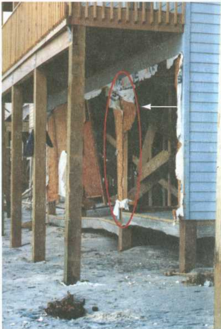
Figure 2-26 Exterior sheathing of breakaway wall spanned piling. Note torn sheathing (arrow).
