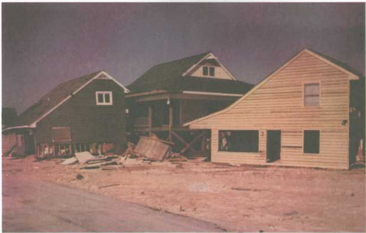
Figure 2-19 Example of extreme impact — two houses floated and pushed into another house.
