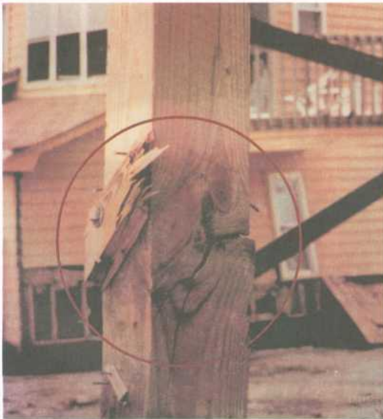
Figure 2-20 Example of broken piling. The piling broke at the location of several knots (circle), where cross-bracing was attached (note remaining bolt and piece of bracing).
