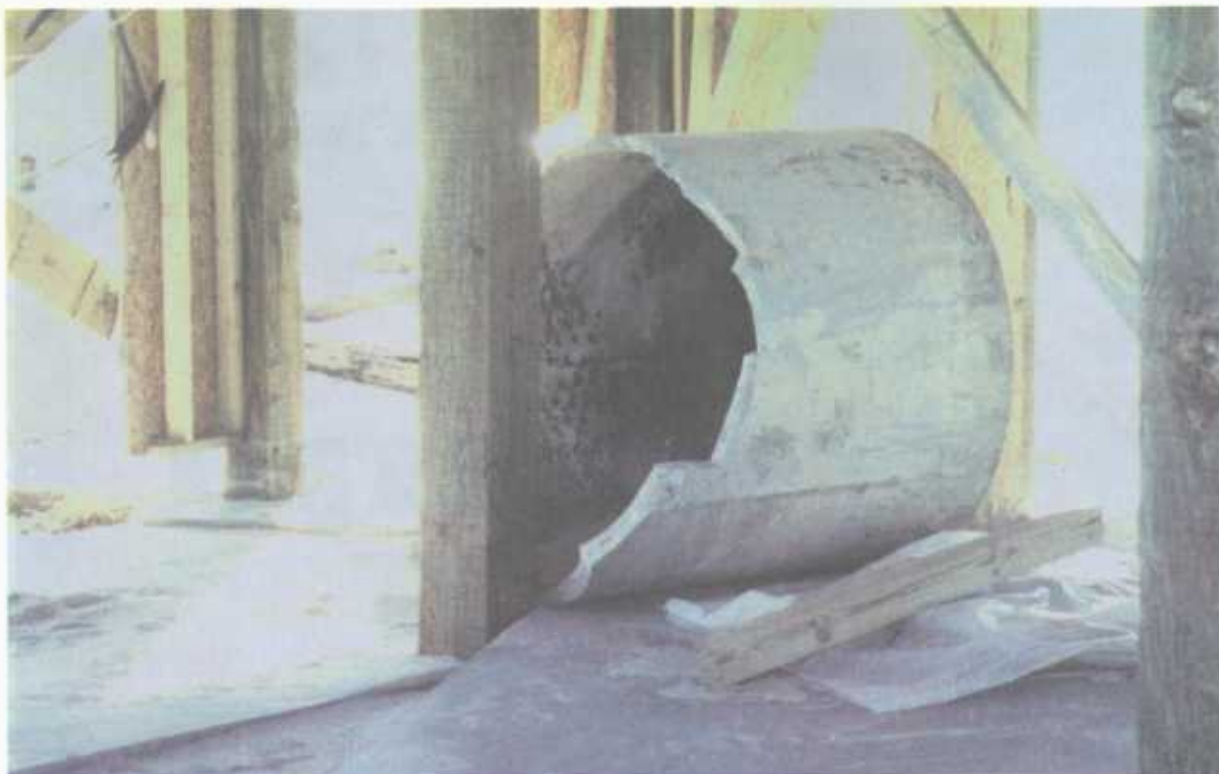
Figure 2-17 Precast concrete ring section of septic tank became waterborne debris, impacting building foundation members.
