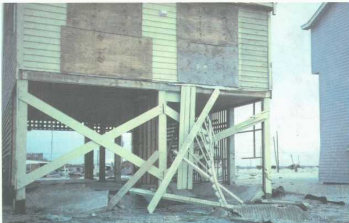
Figure 2-18 Impact of debris from a damaged deck appeared to have broken cross-bracing.
