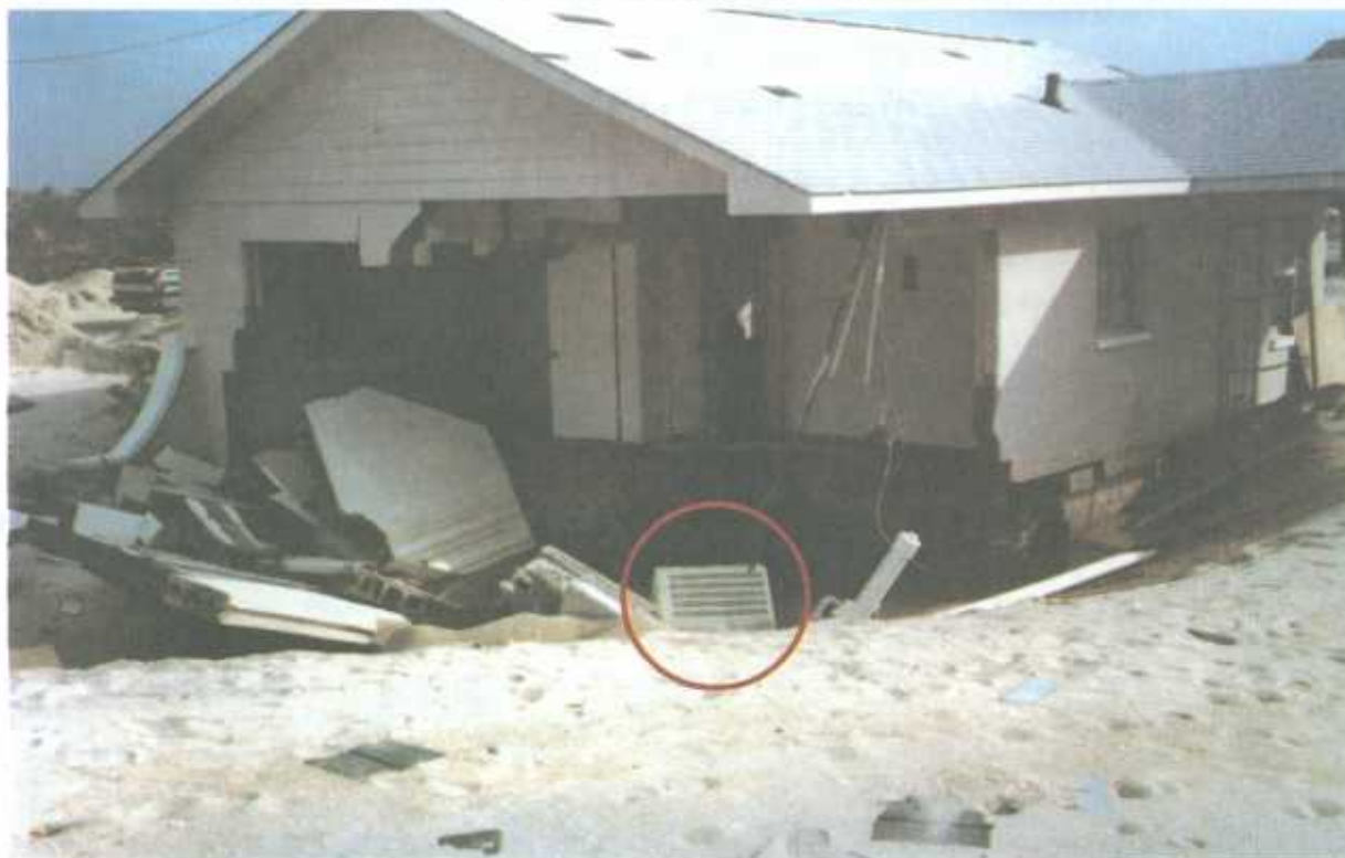
Figure 2-23 Catastrophic failure of landward building constructed on masonry wall and slab-on-grade foundation. Failure resulted because obstruction of flow by building caused extensive scour. Note compressor collapsed into scour hole.
