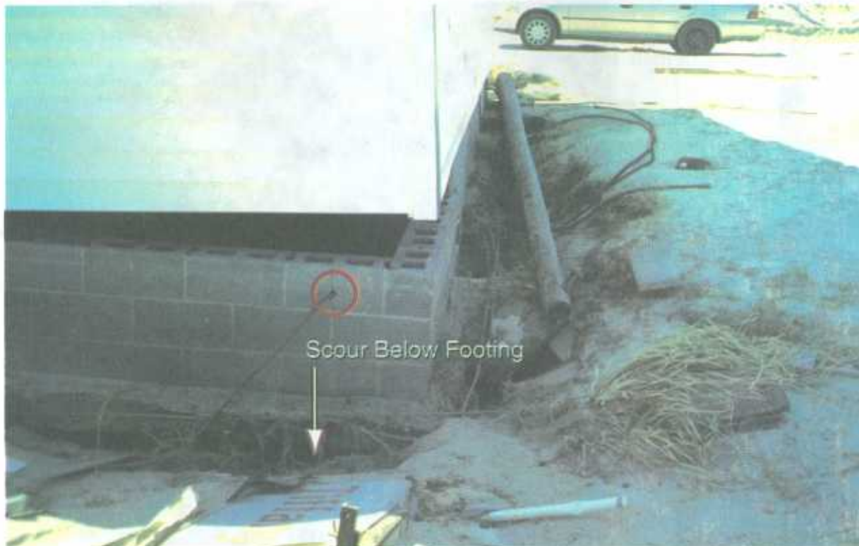
Figure 2-22 Collapse of footing and foundation wall under elevated wood-frame building. Collapse resulted because obstruction of flow by building caused scour to extend below the bottom of the footing (arrow). Note propane gas line (circled) extending through foundation wall.
