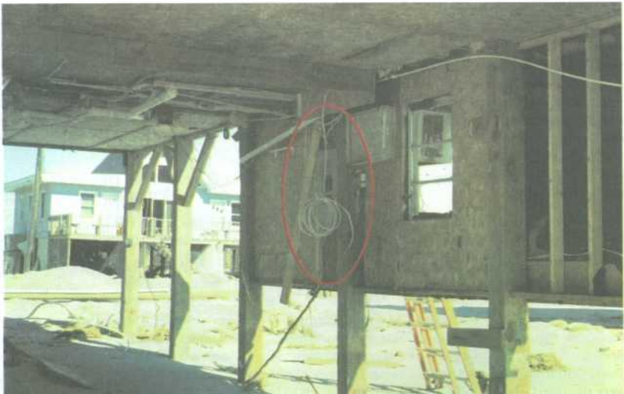
Figure 2-36 Example of utility component (electric panel box) installed on a breakaway wall panel.
