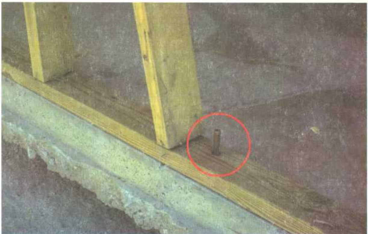
Figure 2-28 Use of anchor bolts through the sill plate of a breakaway wall is improper. Even though this bolt does not have a nut and washer, it prevented the wall from breaking away laterally.
