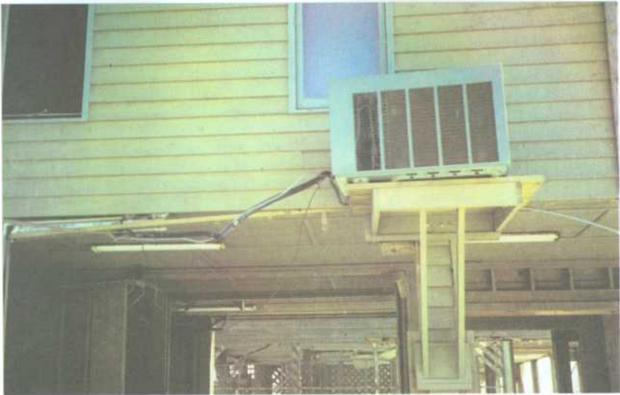
Figure 2-34 Although the air conditioning/heat pump compressor platform on this oceanfront house was adequately elevated with cantilever bracing, the compressor was almost pushed off the platform by wind because of the lack of the necessary attachment.
