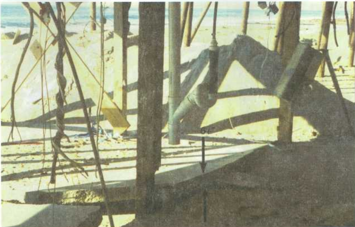
Figure 2-30 Example of unnecessarily thick slab.
