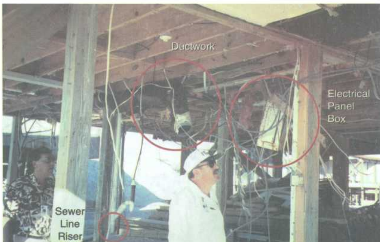
Figure 2-38 These utility components (wiring, electric panel box, ductwork, and sewer line) were installed adjacent to breakaway wall panel and were damaged when the walls broke away. Note broken sewer line riser pipe on seaward side of piling.
