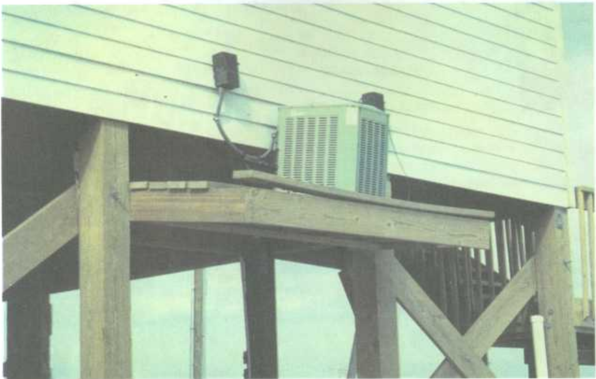
Figure 2-35 Air conditioning / heat pump compressor platform leaning because scour caused loss of two supporting posts.
