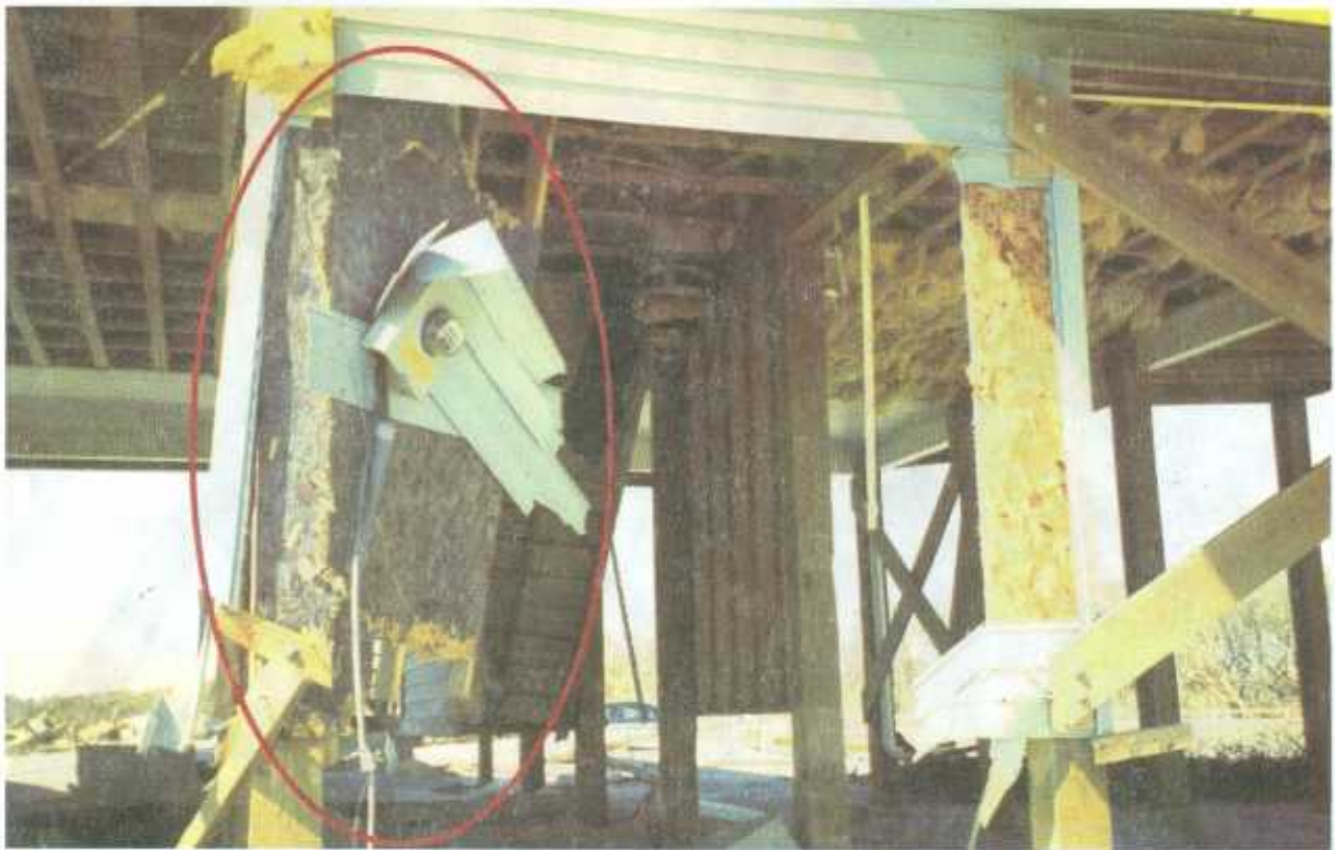
Figure 2-27 Breakaway wall panel failed to function as designed because continuous sheathing was installed across pilings. No structural damage was observed; however, note damage to utility components installed on breakaway wall panel.
