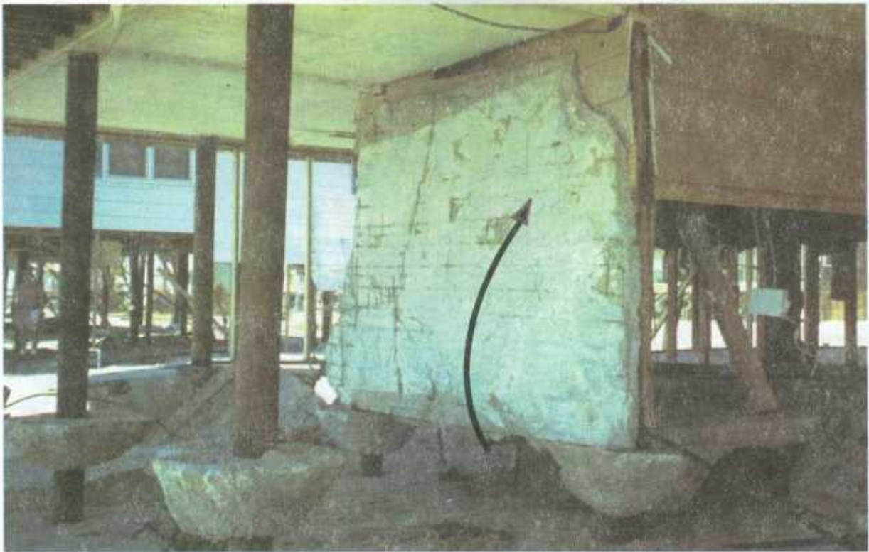
Figure 2-31 Concrete slab-on-grade flipped up, probably by wave action, came to a rest against two foundation members, generating large, unanticipated loads on the foundation. Note slab is supported on concrete collars around piles and contains wire mesh.
