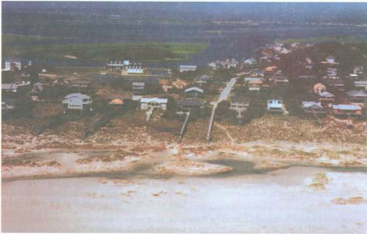
Figure 2-47 As shown by this post-Fran photograph taken at Emerald Isle, North Carolina, proper elevation and setback from the oceanfront in conjunction with substantial protection afforded by dunes resulted in little or no flood damage to the oceanfront row of buildings.
