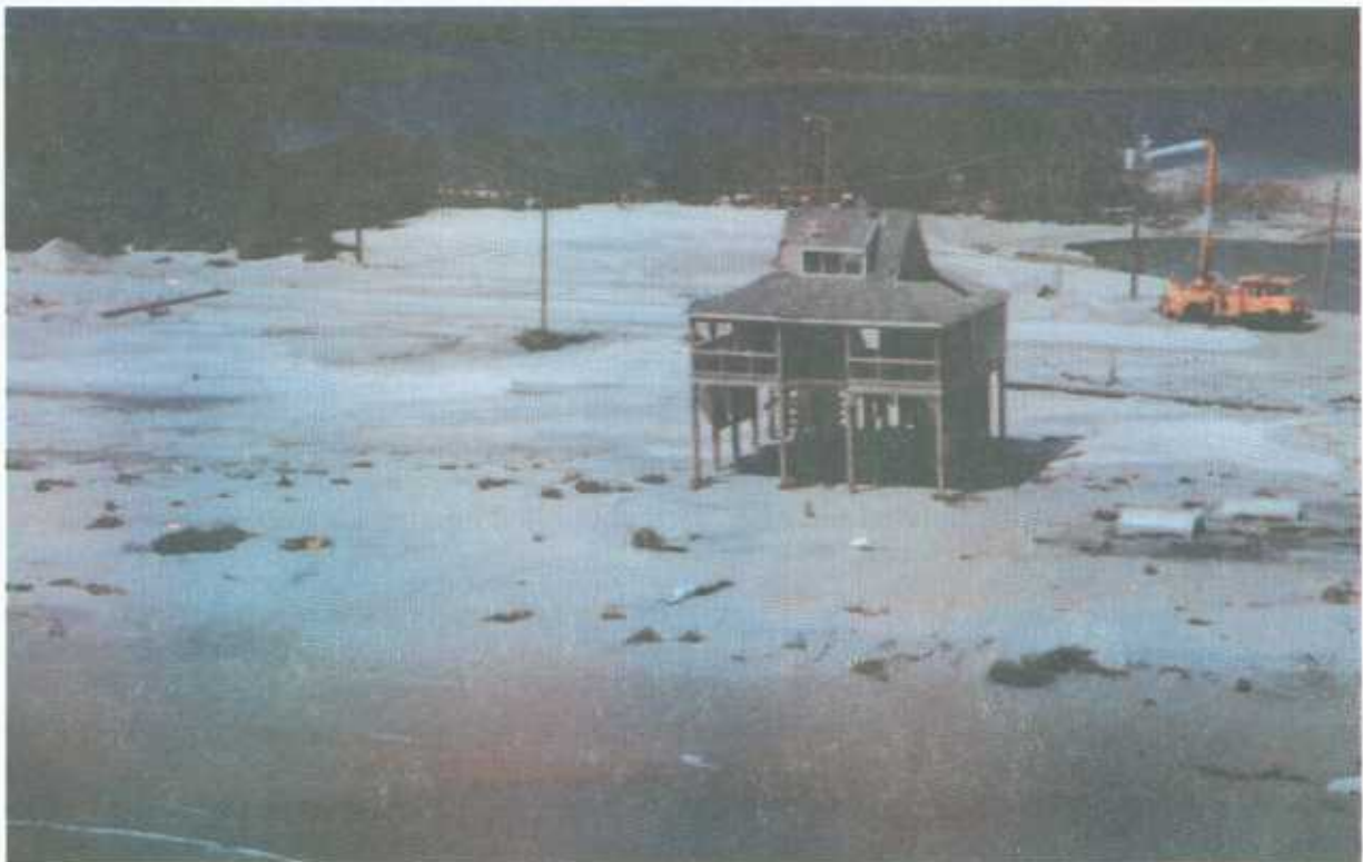
Figure 2-46 While this house experienced 6 feet or more of vertical erosion and scour, as well as the loss of breakaway wall panels, the foundation and superstructure performed as designed.
