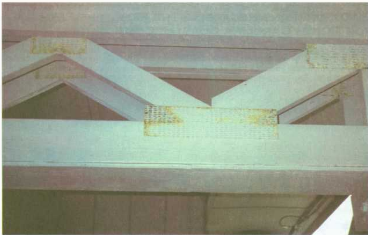
Figure 2-44 Corrosion of galvanized floor truss plates was observed in many buildings. Note that painting does little to slow the process of corrosion in coastal environments
