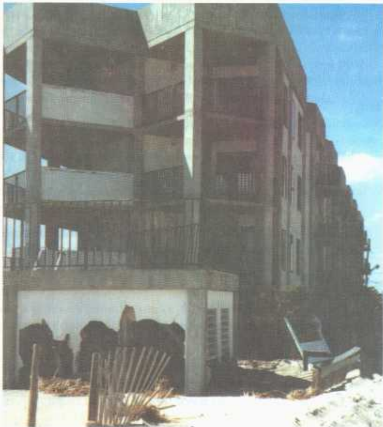
Figure 2-47 As shown by this post-Fran photograph taken at Emerald Isle, North Carolina, proper elevation and setback from the oceanfront in conjunction with substantial protection afforded by dunes resulted in little or no flood damage to the oceanfront row of buildings.
