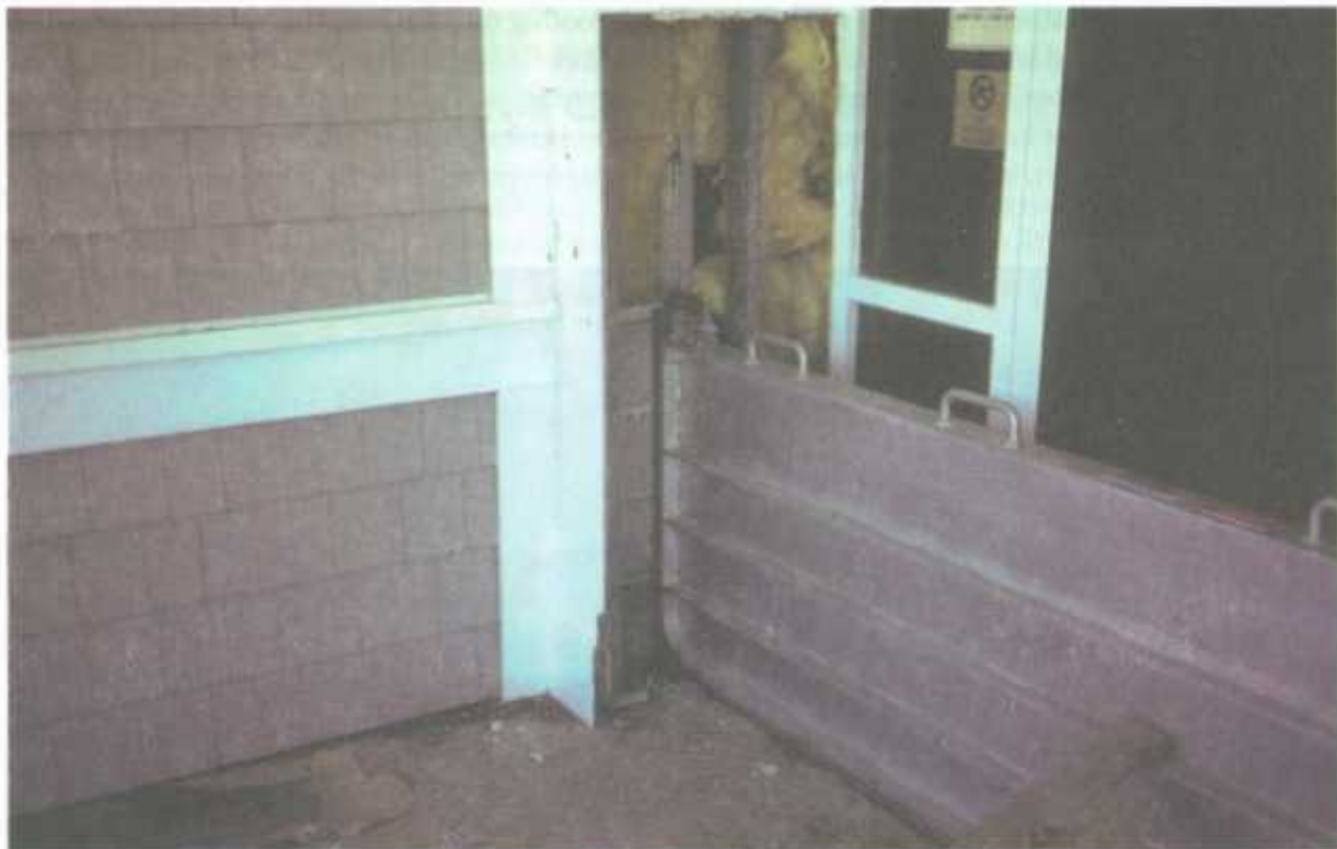
Figure 2-40 Engineered flood shield installed over opening to large dry floodproofed commercial building.
