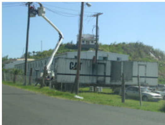
Photo 5 1.5 MW Unit in Lance Aux Epines
