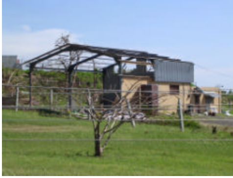
Photo 12 Total Collapse of Walls of Store Equipment Building for PSIA
