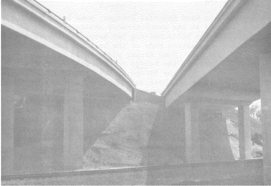
Fig. 5.5 Ward Memorial Boulevard bridges. View looking south towards southern abutment.
