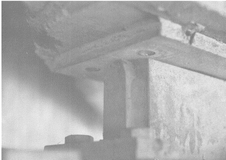
Fig. 5.8 Close-up of rocker bearing showing remnants of sheared keeper plate bolts at top.
