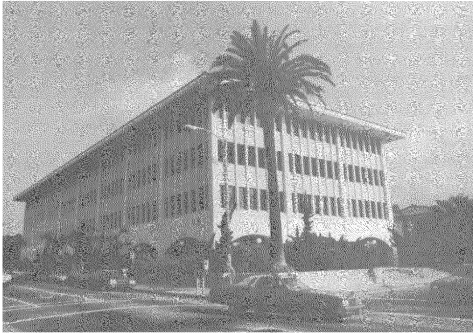
Fig. 7.1 Santa Barbara County Administration Building, a reinforced concrete rigid frame structure.
