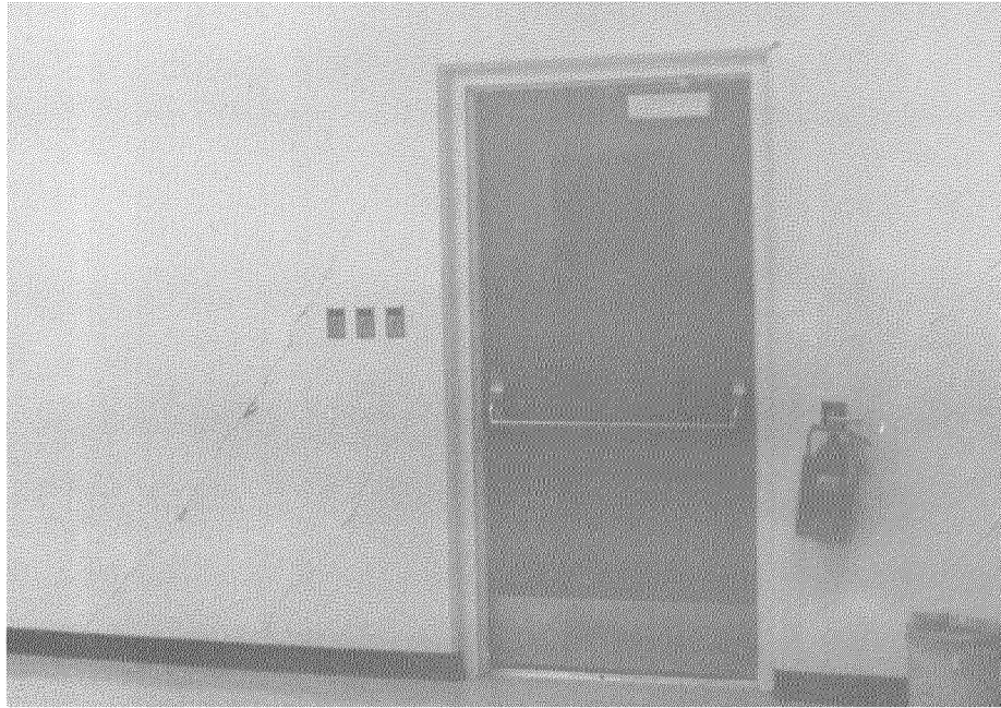
Fig. 7.29 Diagonal cracks in east-west shear wall in first story of Engineering Building, UCSB.
