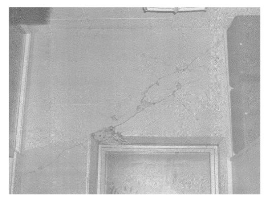
Fig. 7.42 Cracks in shear wall over doorway at west end in first story of Administration Building, Delco Electronics facilities.
