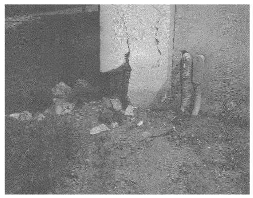
Fig. 7.46 Cracking and spalling of columns at southwest corner of Research and Development Building, Delco Electronics facilities.
