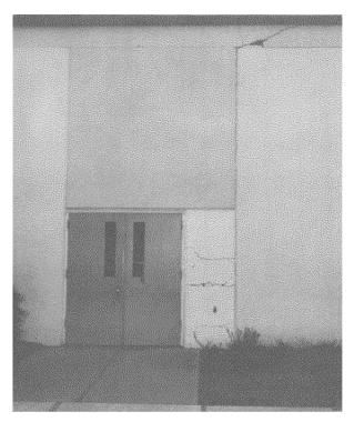
Fig. 7.45 Cracks at joints between panels and doors, Research and Development Building, Delco Electronics facilities.
