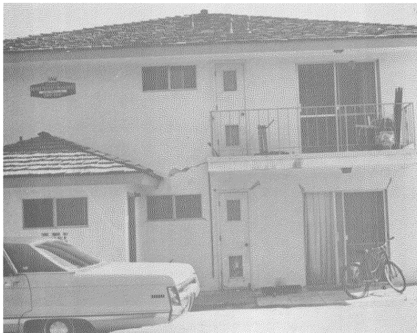
Fig. 7.51 Cracks in exterior plaster walls of two story residential building in Isla Vista.
