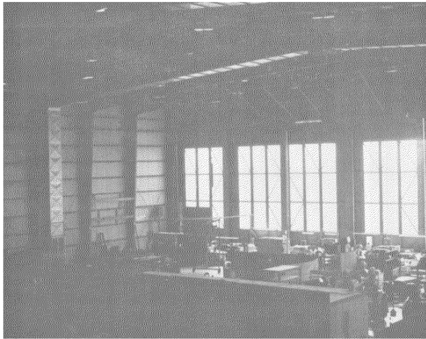
Figure 7.66 Interior of large hangar at facilities of Aero Spacelines, Inc., showing large sliding doors and damaged steel bracing which angles up to the roof from the rail at top of doors
