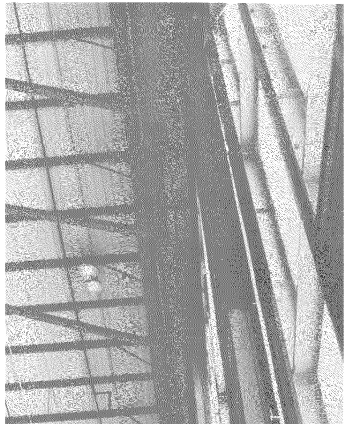
Figure 7.67 Close up from directly under damaged steel bracing of sliding doors shown in Fig. 7.66. Note separation of rail and bracing in center of picture
