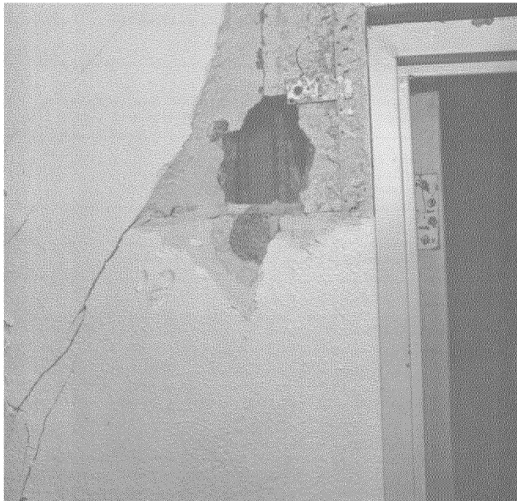
Fig. 7.22 Face of concrete block removed to expose ungrouted reinforcing steel, shear wall in Anacapa Residence Hall.
