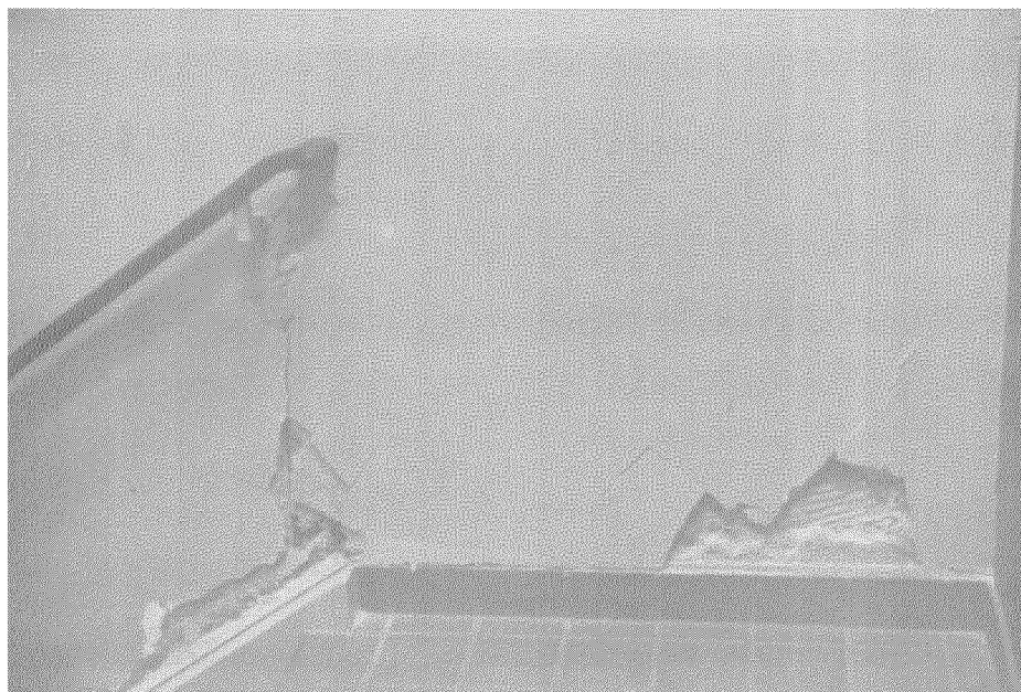
Fig. 8.7 Cracks in plaster wall of Santa Barbara County Administration Building.
