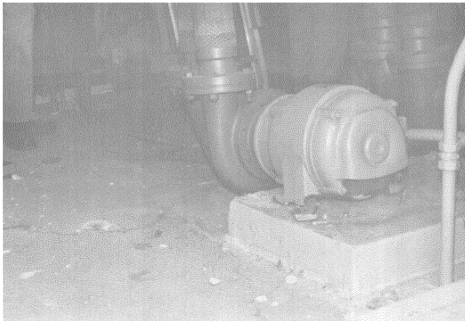
Fig. 8.11 Broken mounting base of hot water pump on top of Library III Building, UCSB.
