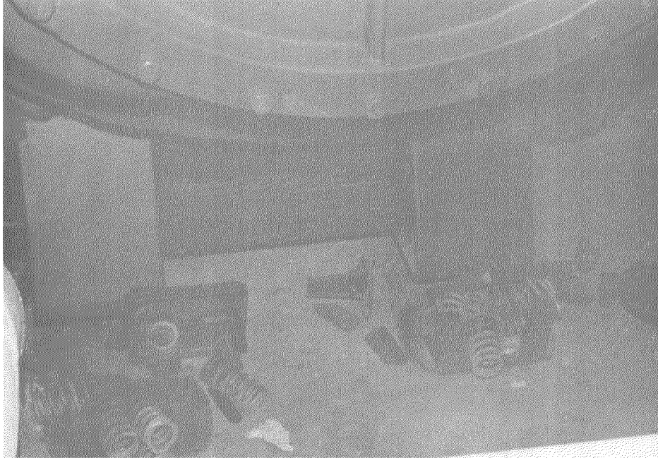
Fig. 8.10 Close up of damaged supports at back of chiller (Fig. 8.8).
