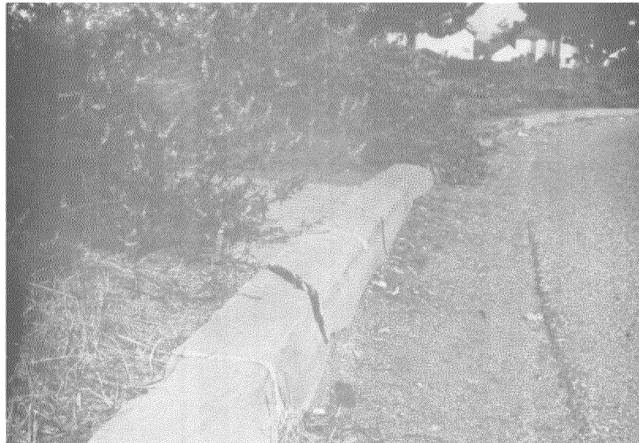
Fig. 9.10 Close up of curb push out shown in Fig. 9.9. (View from south.)
