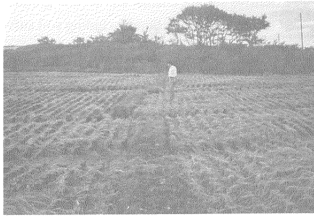
Photo 9 Fissures and Sharing of Ground Appeared in Kabutono Area ( Area B. see Fig. 4, View to Crescent Lake taken at September 1993)
