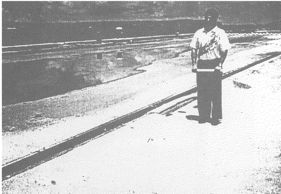
Figure 5: Differential settlement between the pile-supported crane railing and the adjacent filled areas
