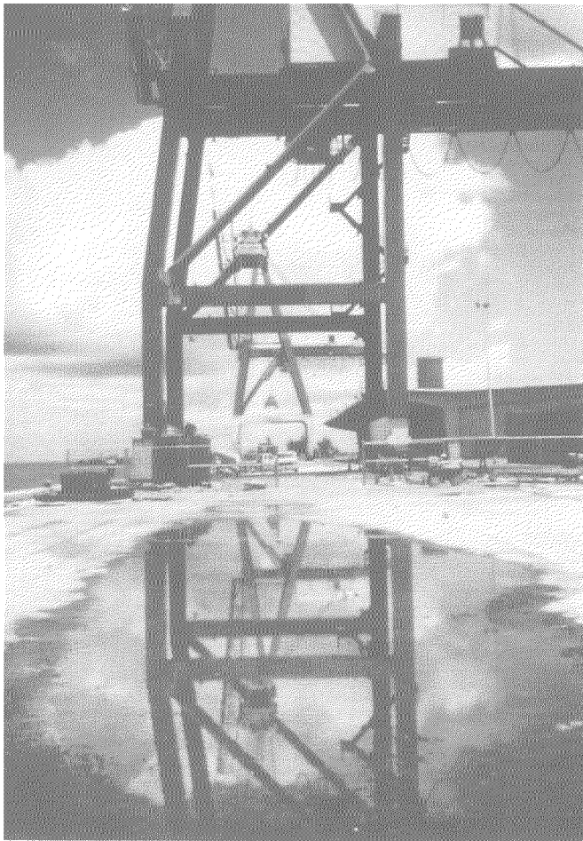
Figure 6: Settlements of up to 18 inches disrupted the surface drainage at the commercial port facilities
