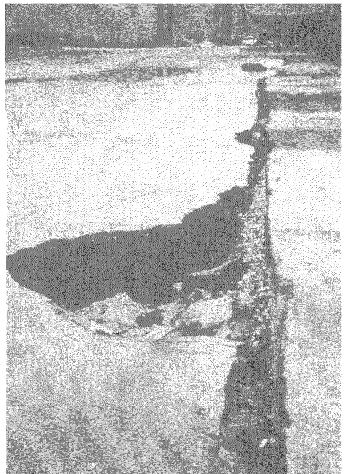
Figure 7: Lateral movement and cracking of the pavement, commercial port facilities
