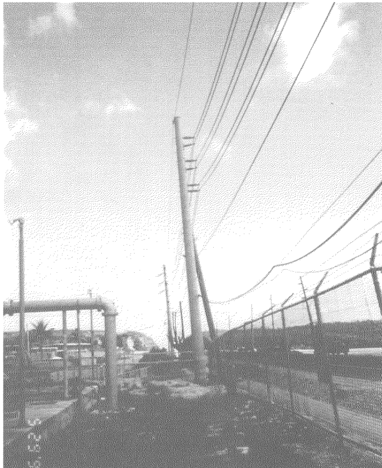
Figure 11: Leaning of the power poles caused by lateral spreading at the Piti Electric Power Plant
