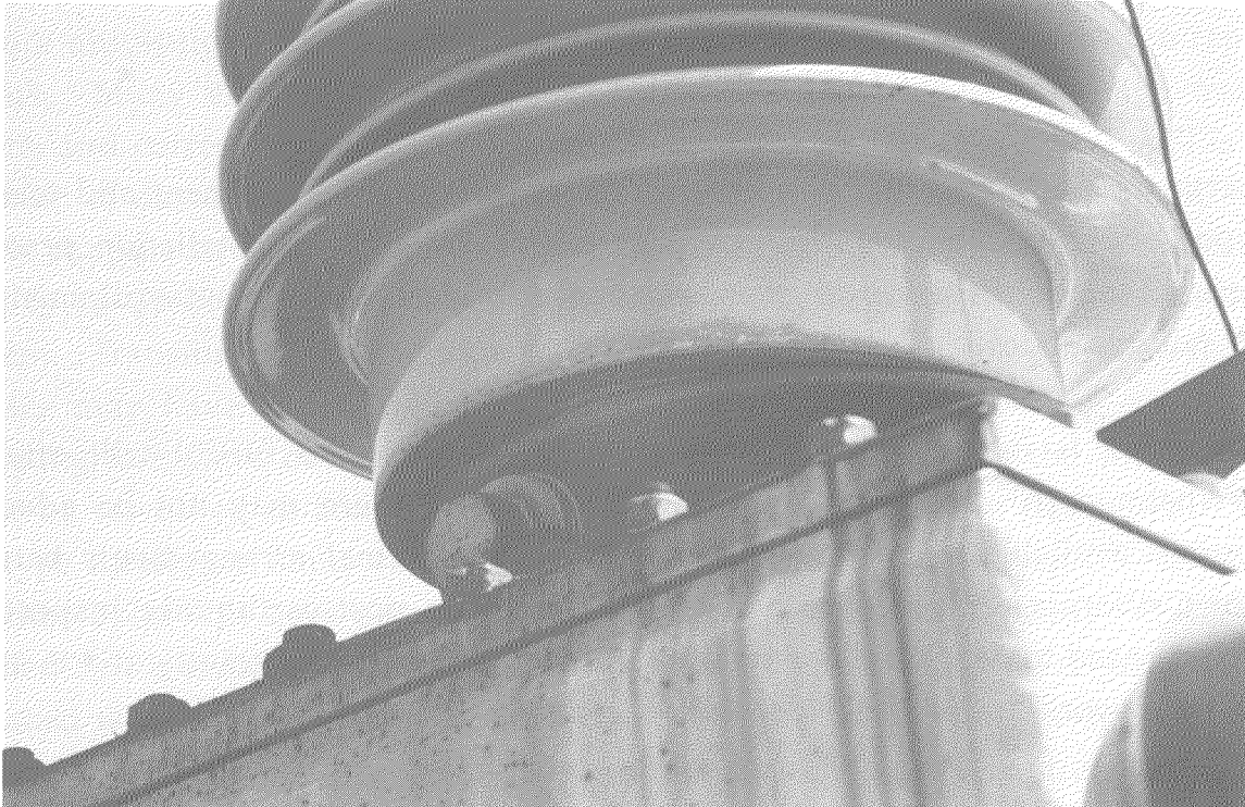
Fig. 1 Shifted Transformer Bushing
