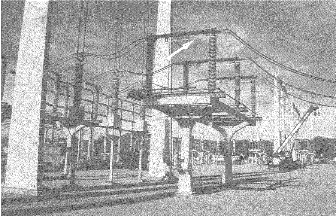
Fig. 2 Rope Used To Temporarily Place A Disconnect Switch Back Into Service.
