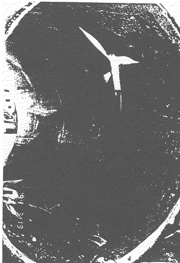
Photo 1 Damage to Granada Trunk Line
