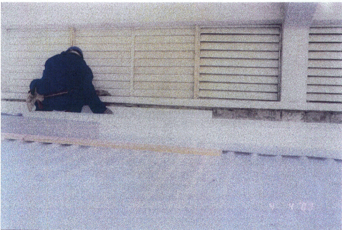
Fixing Flashing (CHEST WING)
