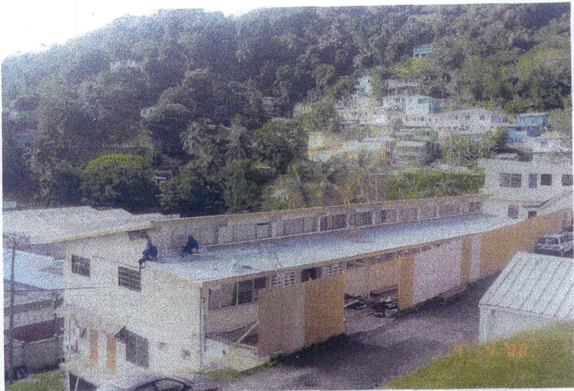
Chest Wing Building, Hoarded Off
