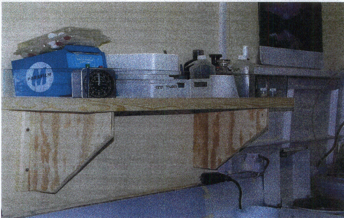
Note 4" high plexiglass protection to shelves
