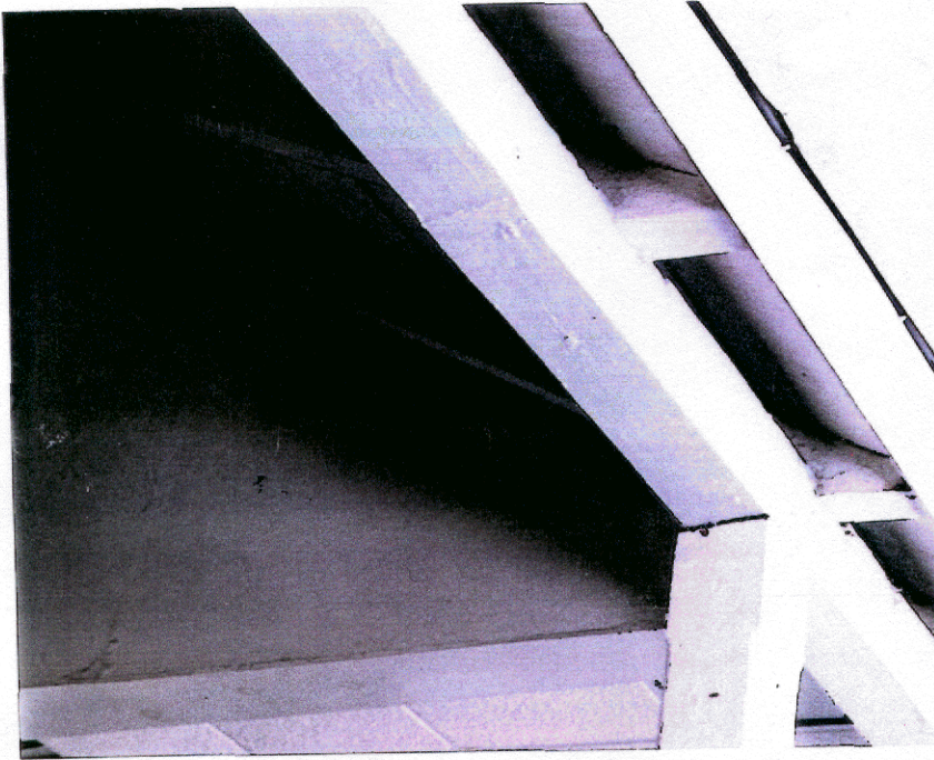
PHOTO 31 BEAM-COLUMN UNION IN CORRIDORS OF BUILDINGS A, B AND D
