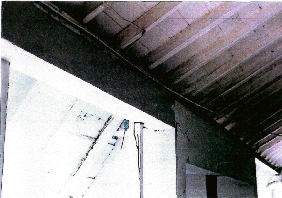
PHOTO 44 DAMAGE TO BEAMS IN EASTERN CORRIDOR OF BUILDINGS B AND D
