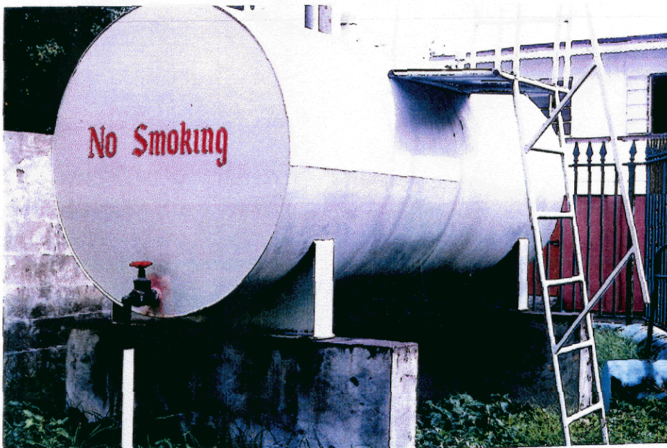
PHOTO 46 DETAIL OF GASOIL TANK SUPPORTS
