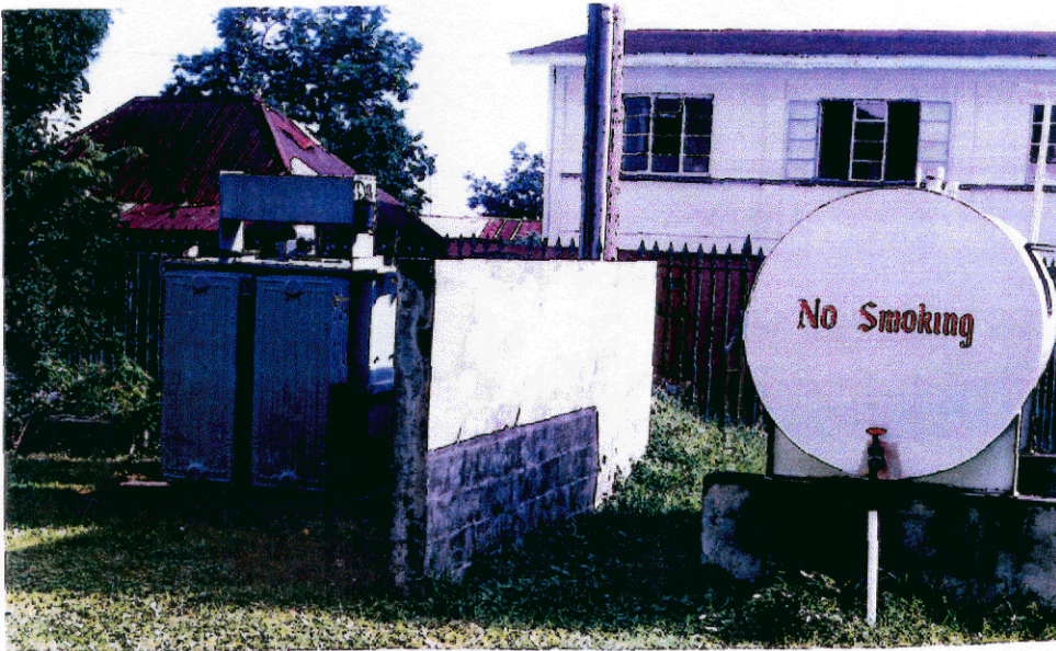
PHOTO 45 HIGH VOLTAGE TRANSFORMER, FIRE-PREVENTIVE WALL AND GASOIL TANK
